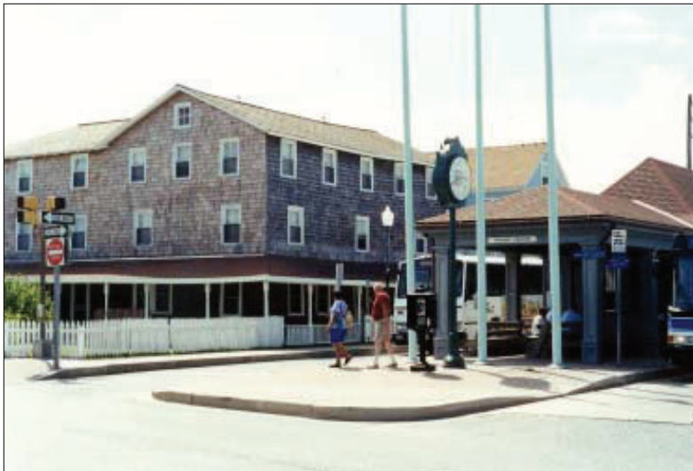
The Ocean City Transit Center in Worcester County enhances the architectural character of the downtown area and serves visitors from a convenient location near the boardwalk. [Photo by Kip Van Blarcom]
