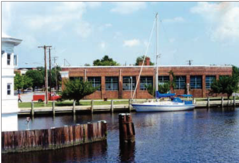
This former automobile garage in Pocomoke City, Worcester County, will soon be transformed into the Pocomoke River Discovery Center, a significant new attraction. [Photo by Kip Van Blarcom]
