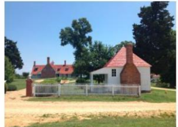
Sotterley Plantation gatehouse project. Photo provided by Nancy Easterling.
