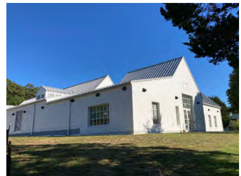
The newly-renovated MAC Lab exterior.
