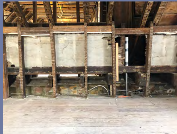
The original floor level and plaster wall sitting about two feet above the existing floor. Note the black-painted baseboard and pieces of the intact plaster wall above.
