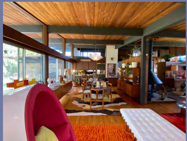
The interior of the Hirsch Residence, featuring oak floors and stained cedar ceilings with exposed wood rafters. (Source: EHT Tracerics)
