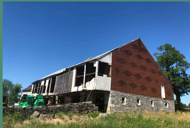
Brick and lumber salvaged from the historic brick pierced-end barn and other outbuildings will be repurposed for new uses.
