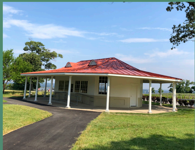
Fort Smallwood Concession Stand after renovation
