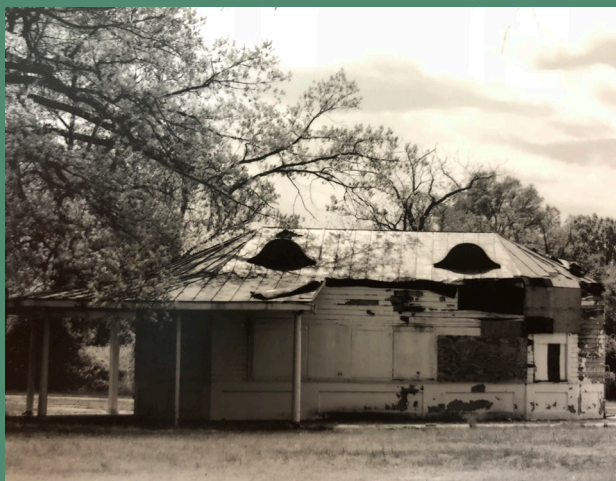
Fort Smallwood Concession Stand pre-renovation
