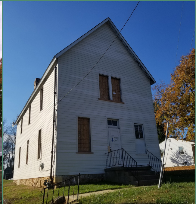
The fellowship hall following the first phase of renovation.
