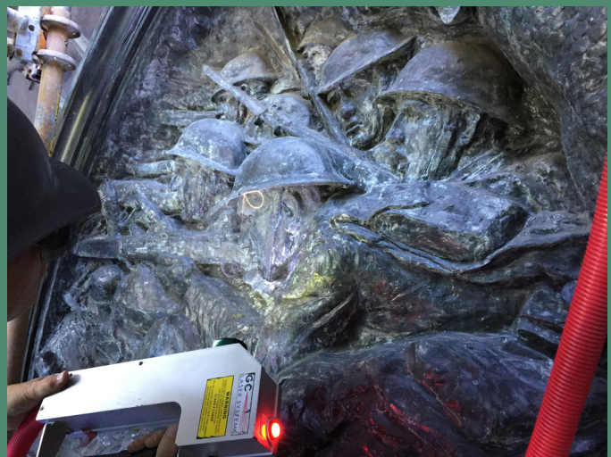
Conservator Andrzej Dajnowski uses laser technology to clean the World War I memorial by Baltimore sculptor Hans Schuler at the Fifth Regiment Armory in Baltimore.
