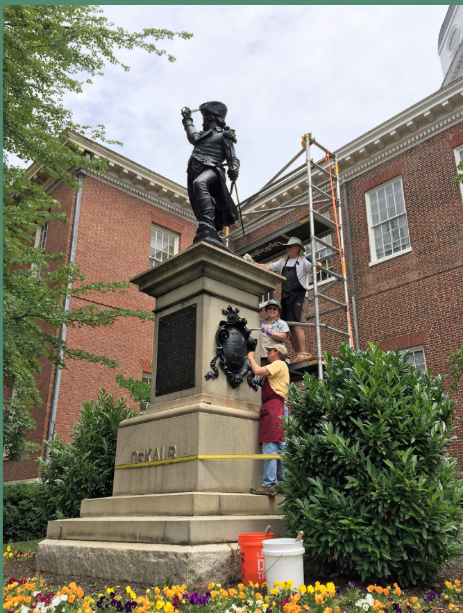
Conservators Howard Wellman, Ronald Harvey and Constance Stromberg wash and renew the wax coating on the Baron de Kalb monument on the State House grounds.
