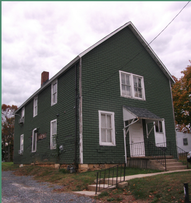
The fellowship hall before work commenced in 2015.
