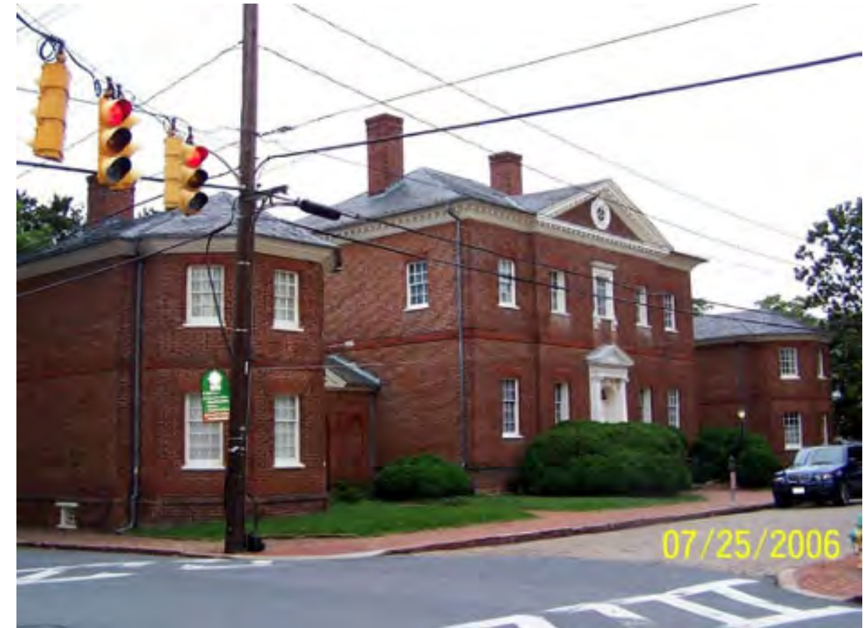
July 25, 2006. Looking southeast.
