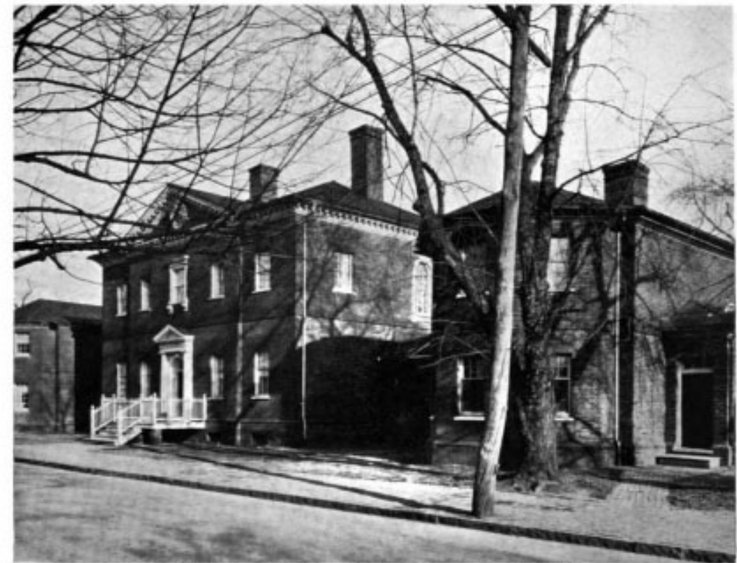
GENERAL STREET VIEW. PORCH AT EXTREME RIGHT IS MODERN WORK.
