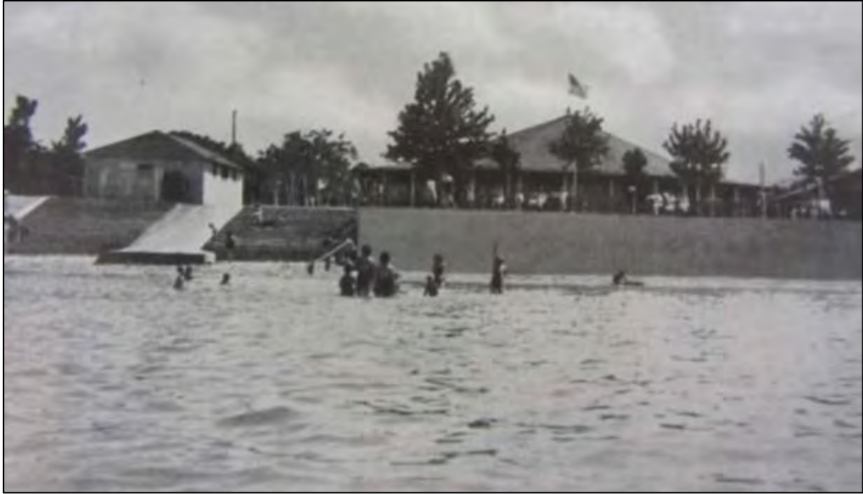
Figure 13– Two of the buildings, along with a seawall can be seen at Kurtz Pleasure Beach in this undated photograph. (Collection of Jack Kelbaugh, reproduced in The Pasadena Peninsula , by Isabel Shipley Cunningham, 127)
