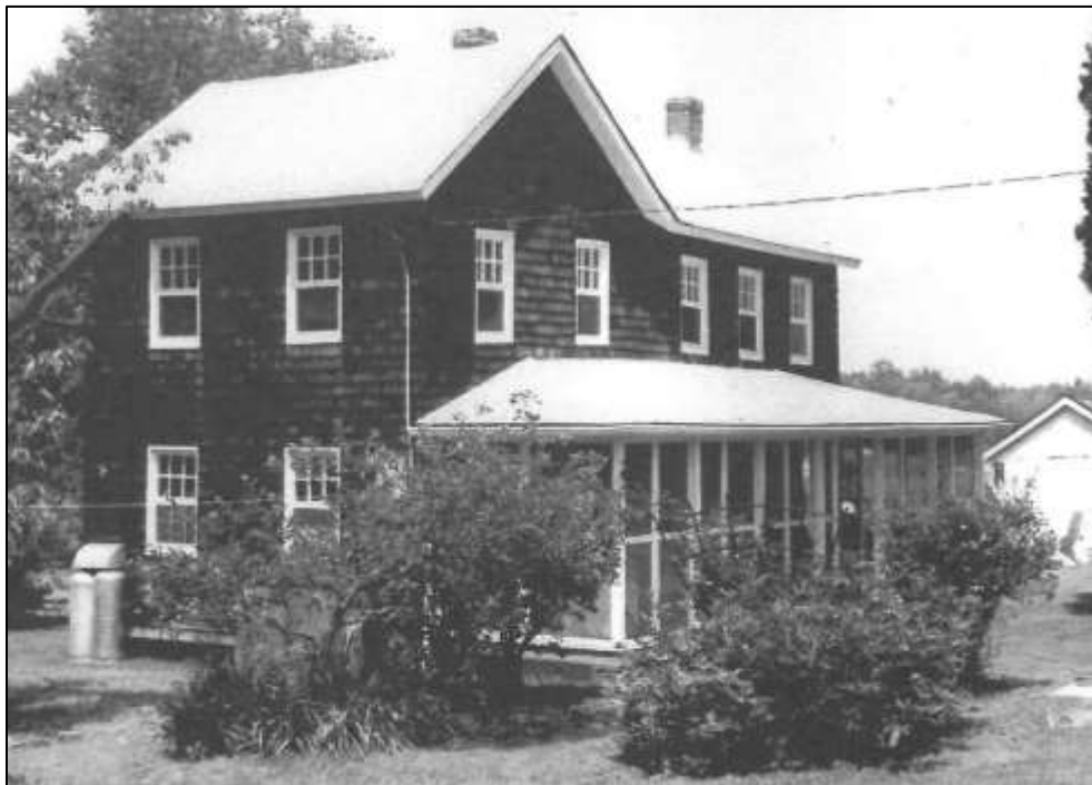
Figure 6 – August Quade and his brother Herman built the three-bay section of this house on the right in 1894. (“August Quade House,” Maryland Inventory of Historic Properties Form AA-2077, July 1987, Maryland Historical Trust website, https://mht.maryland.gov/secure/medusa/PDF/AnneArundel/AA-2077.pdf )
