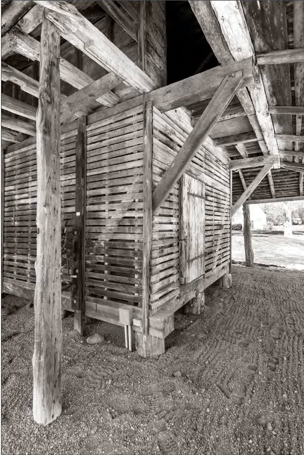
Figure 66. Gapped slats, corn crib, Sotterley (Willie Graham).
