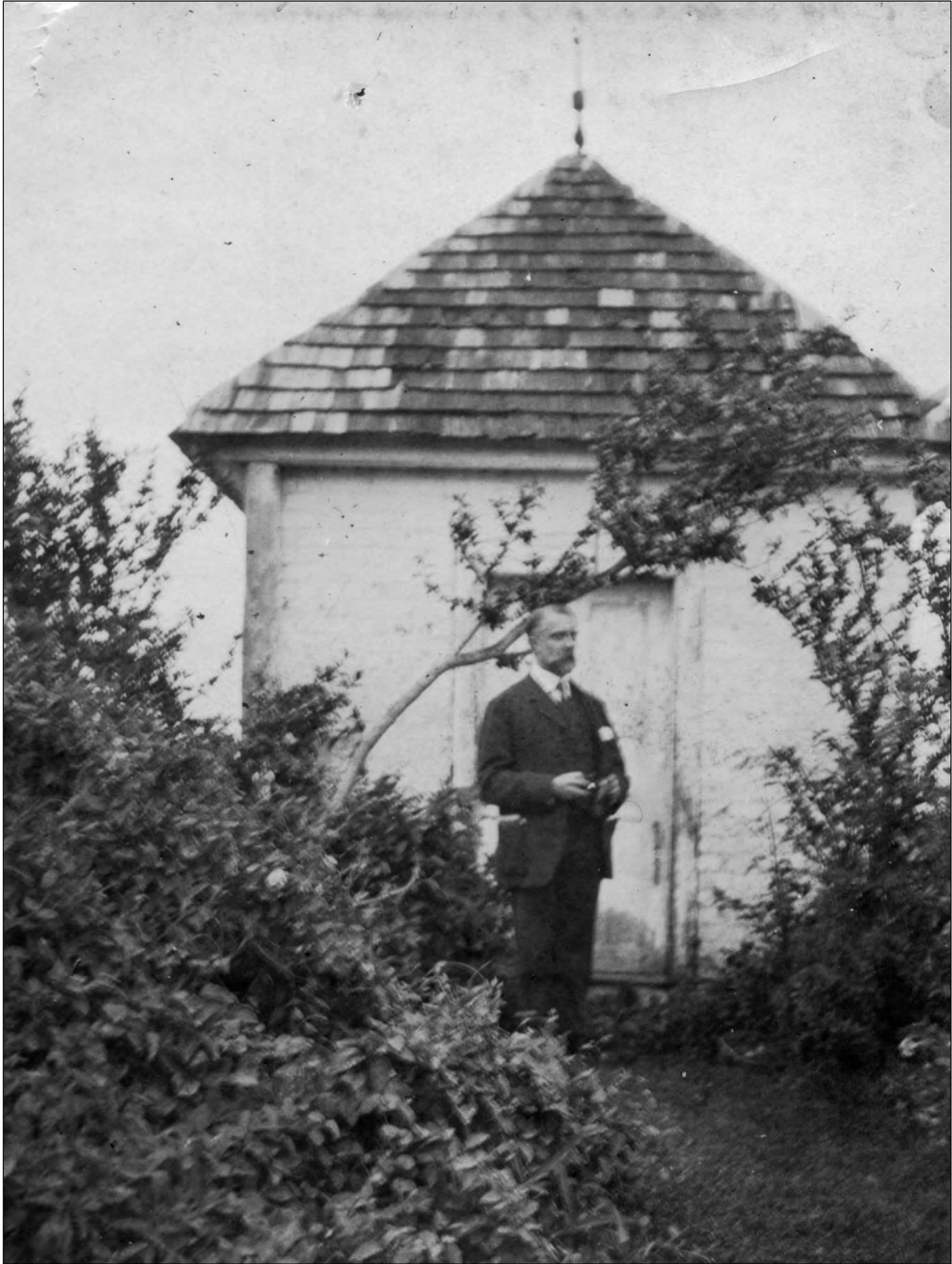
Figure 69. Sotterley privy before restoration, c. 1914 (Historic Sotterley).
