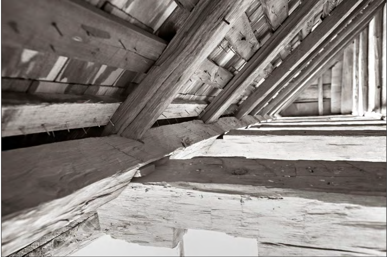
Figure 65. Tilted false plate, corn crib, Sotterley (Willie Graham).
