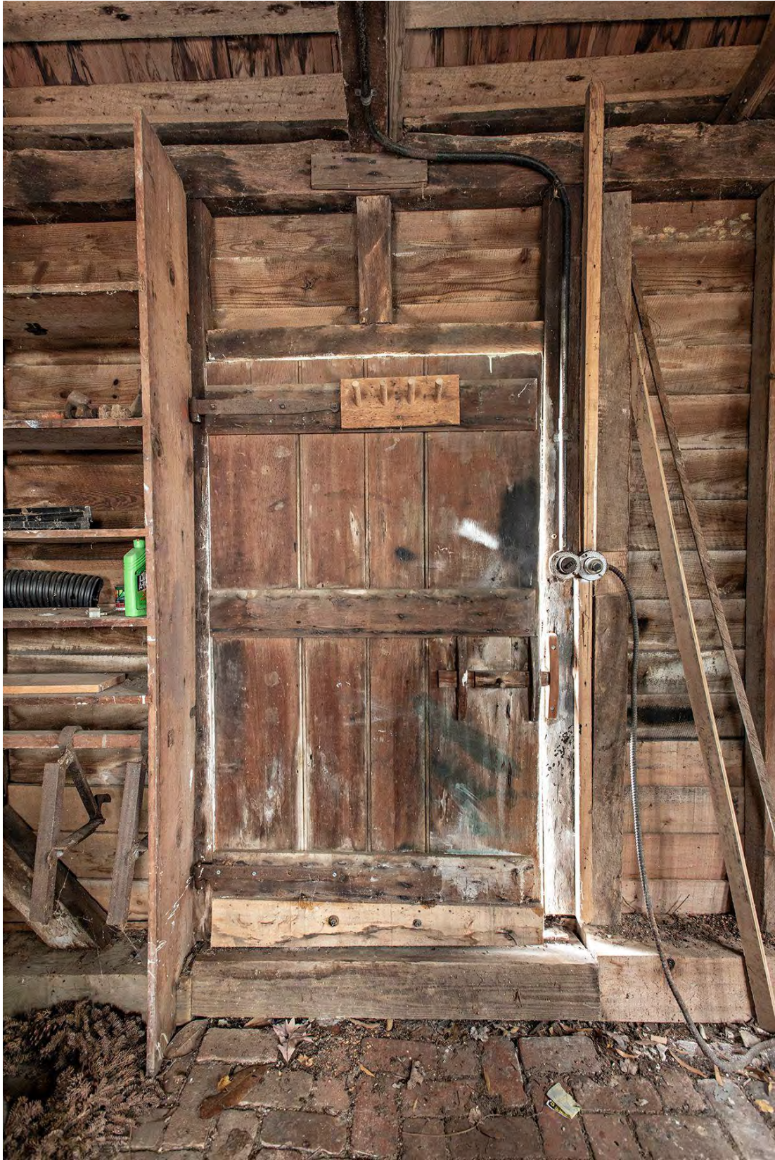
Figure 50. Antique door replacement in the smokehouse, Cremona (Willie Graham).
