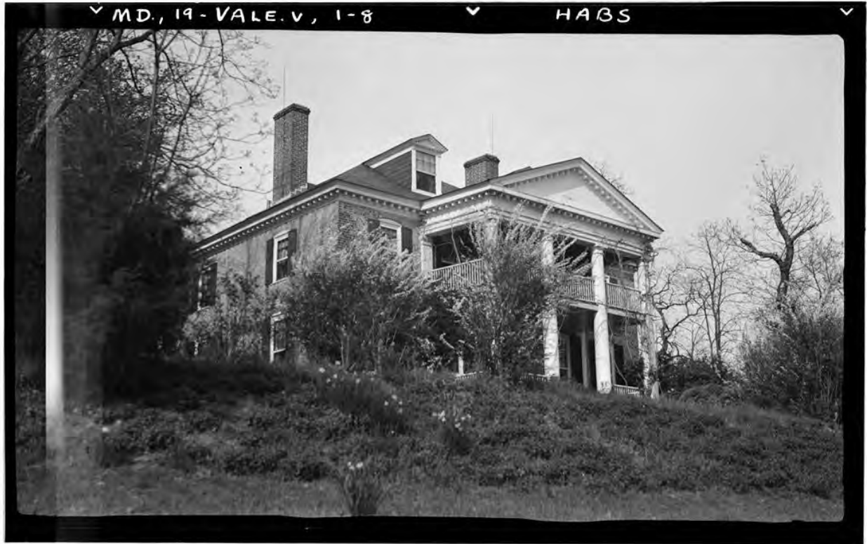
Figure 54. Mulberry Fields, south façade (HABS).
