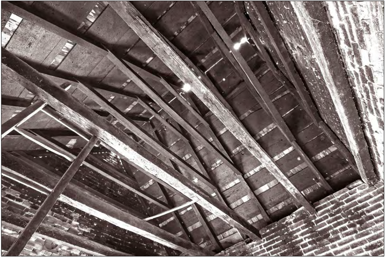
Figure 25. Compton Bassett smokehouse roof framing (Willie Graham).
