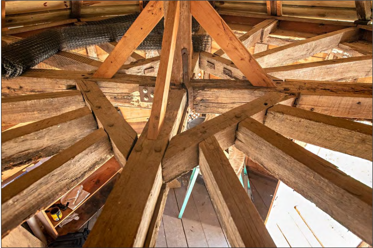
Figure 43. Dairy roof framing, Mount Lubentia (Willie Graham).
