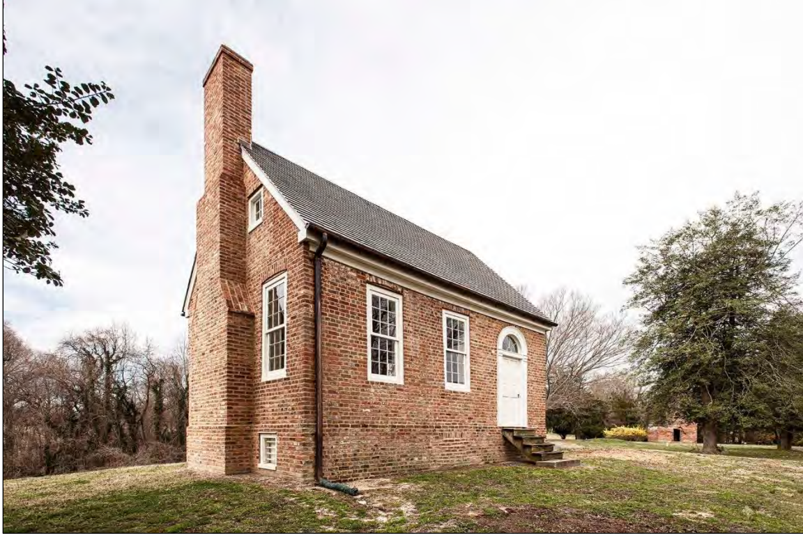
Figure 26. Compton Bassett brick building later converted to chapel (Willie Graham).
