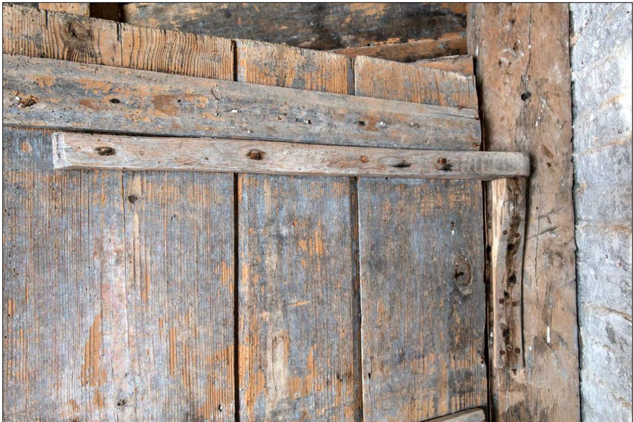
Figure 58. Wooden hinges, board-and-batten door, workhouse/weaving house, Mulberry Fields (Willie Graham).
