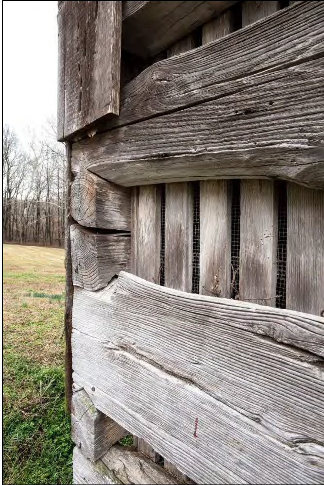
Figure 5. Cedar Hill corn crib, vented walls (Willie Graham).
