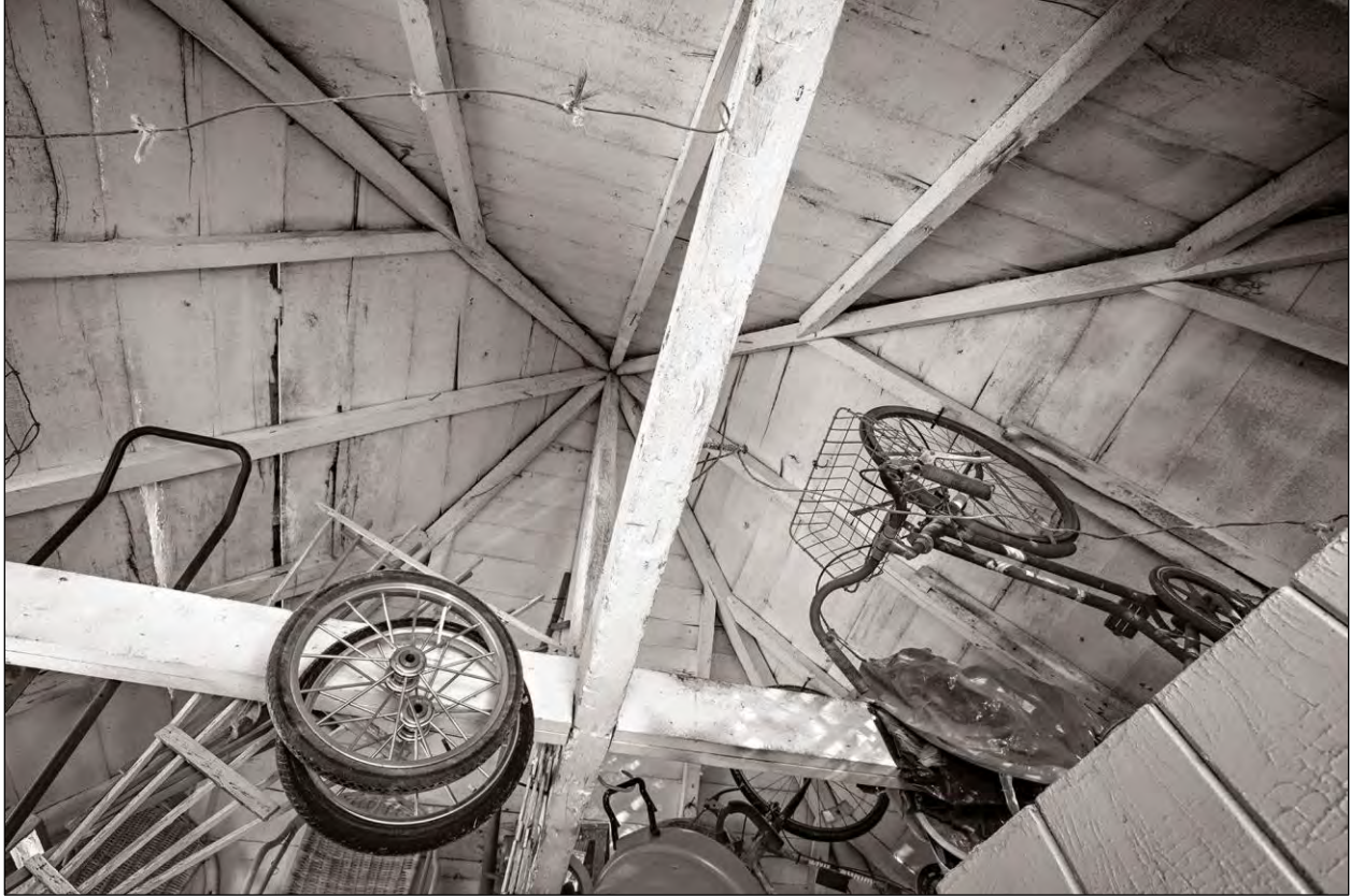
Figure 10. Interior view of the dairy roof, Araby (Willie Graham).
