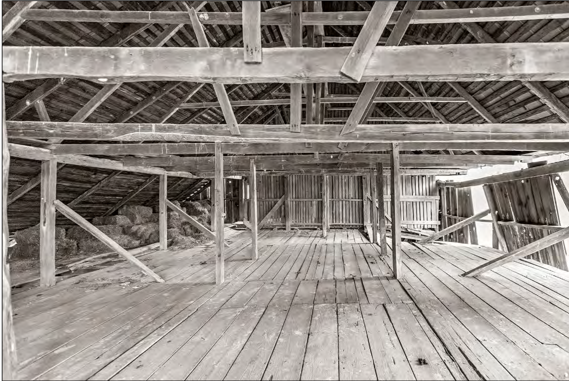
Figure 28. Compton Bassett barn interior (Willie Graham).
