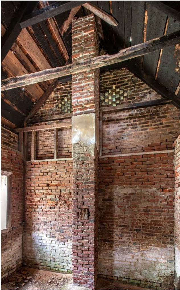
Figure 37. Stove chimney added to rear wall, smokehouse, Poplar Hill at His Lordship's Kindness (Willie Graham).
