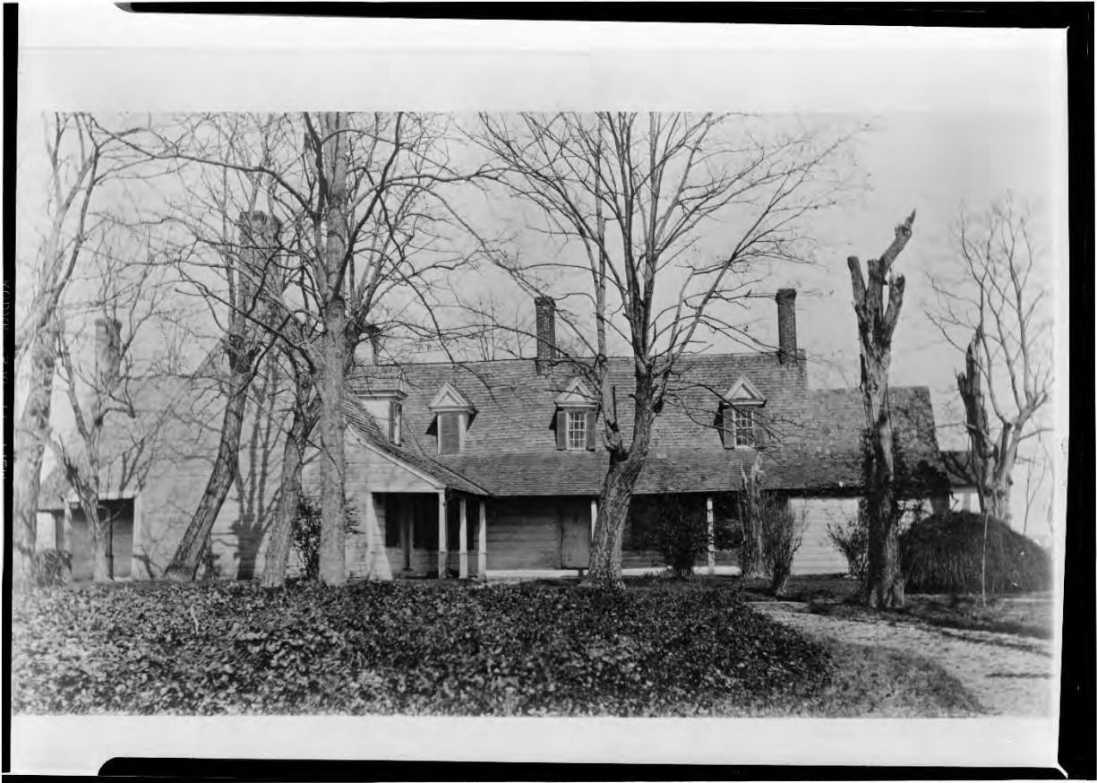
Figure 62. Sotterley before its restoration by the Satterlee family, c. 1911 (HABS).
