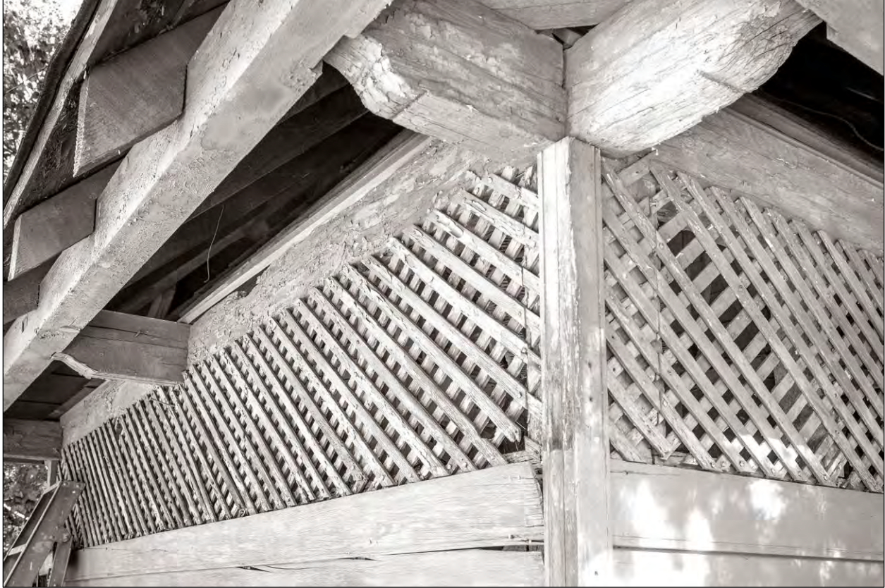
Figure 11. Lattice ventilation, Araby (Willie Graham).
