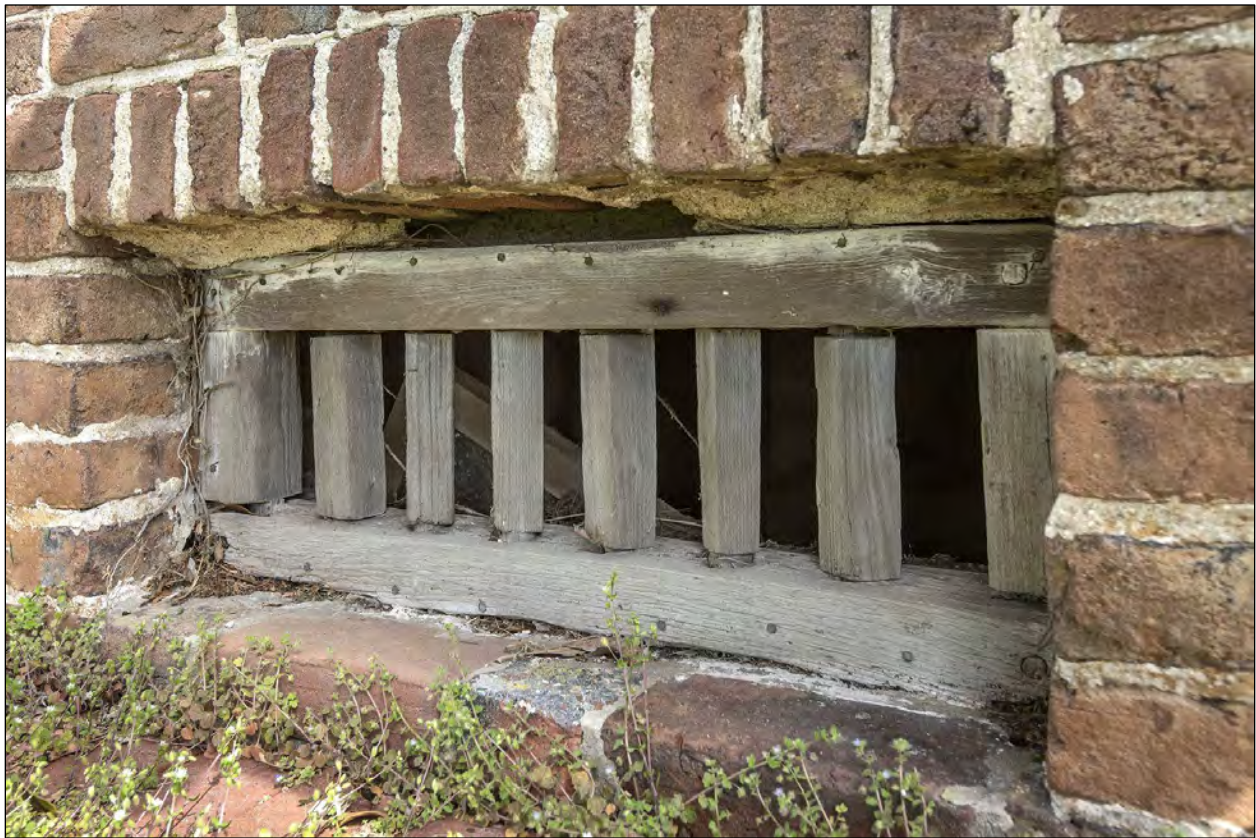
Figure 57. Cellar window vents, workhouse/weaving house, Mulberry Fields (Willie Graham).
