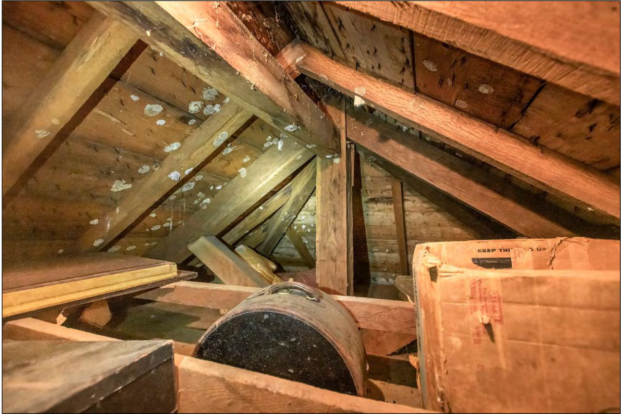
Figure 60. Main house roof, Mulberry Fields (Willie Graham).
