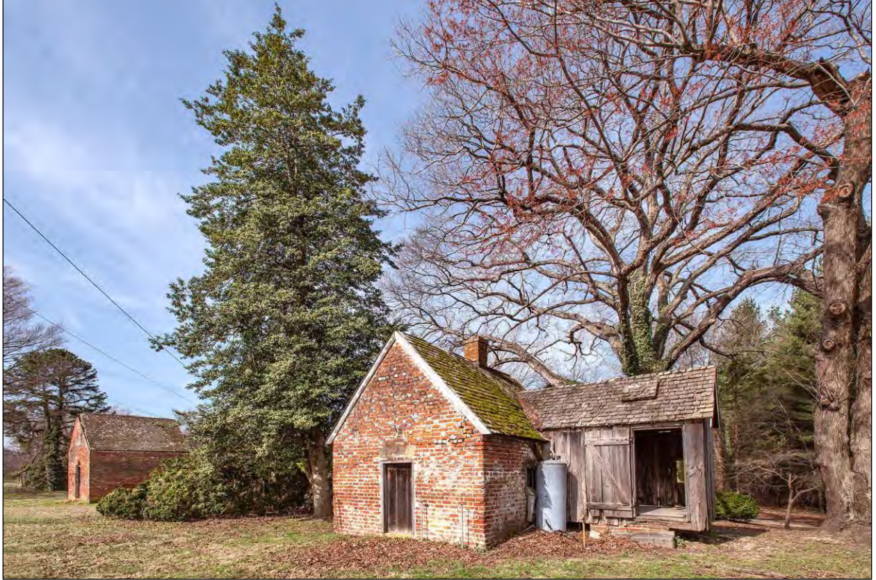
Figure 21. Compton Bassett dairy with the smokehouse to the left (Willie Graham).
