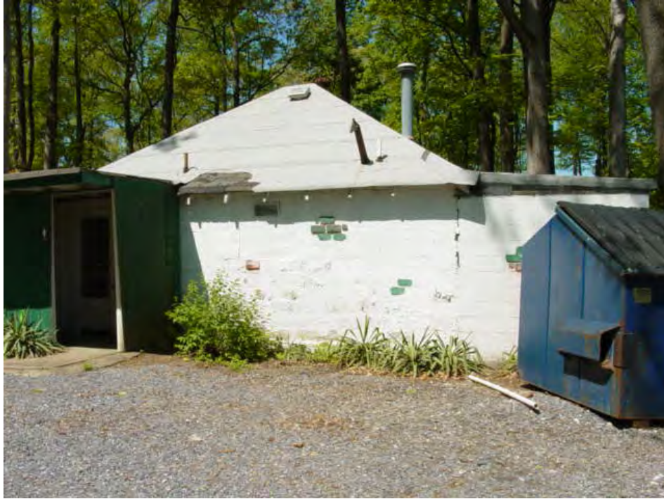
Figure VI-43: The concrete-block, pyramidal-roofed bathhouse that holds the showers and toilets for the cottage dwellers at Spencerville. (Elizabeth Jo Lampl, Montgomery County Historic Preservation Section)
