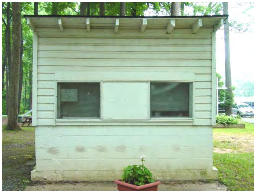
Figure VI-38: The novelty-sided, first aid building at Spencerville, now used by the Christian Youth Crusaders. (Elizabeth Jo Lampl, Montgomery County Historic Preservation Section)
