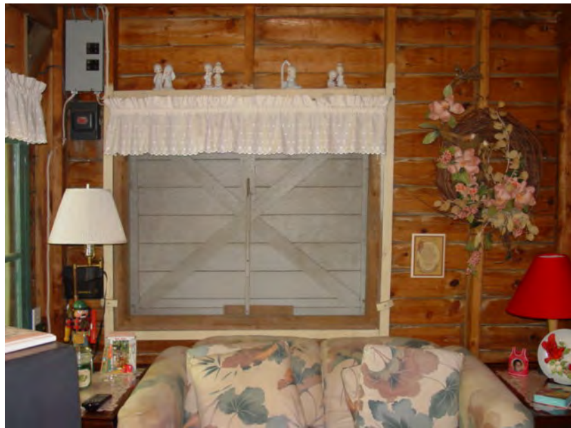
Figure VI-15: Interior of Spencerville cottage showing shuttered and screened window openings, with operable shutters hinged at the top. (Elizabeth Jo Lampl, Montgomery County Historic Preservation Section)
