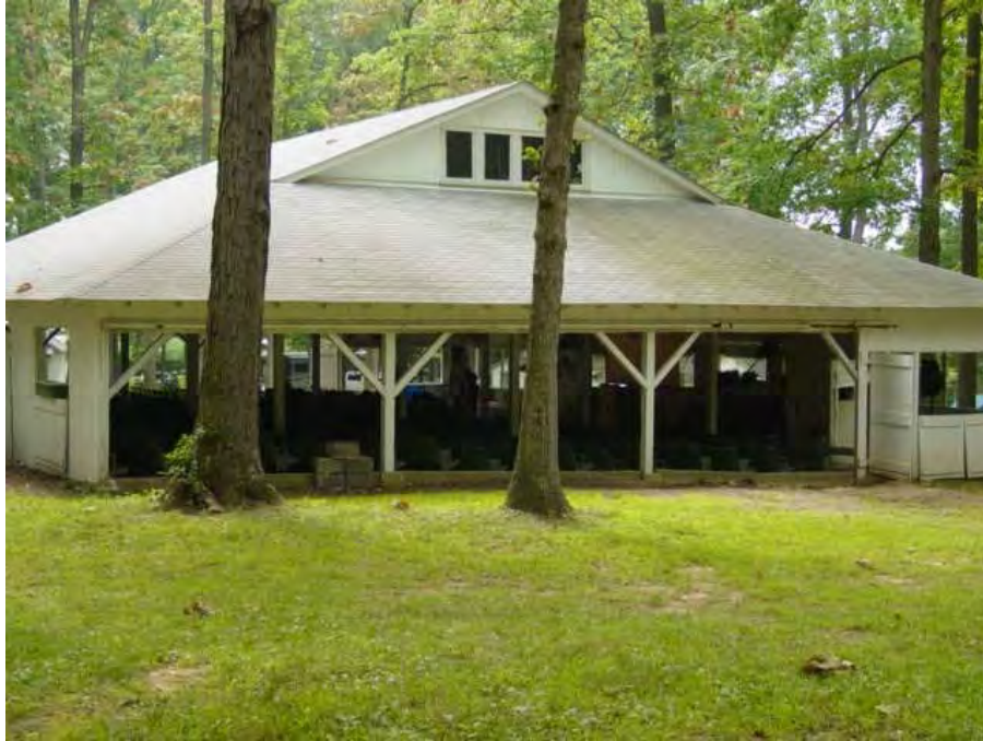
Figure VI-22: The west wall of the Spencerville tabernacle, which originally featured bi-fold doors that operated along a track. The tabernacle is opened up for the July camp meeting. (Elizabeth Jo Lampl, Montgomery County Historic Preservation Section)
