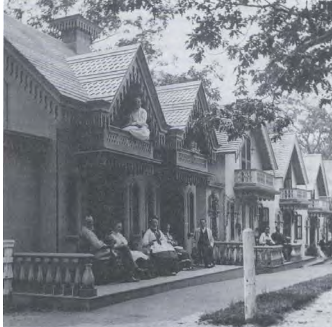
Figure VI-9: The basically uncovered porches of Wesleyan Grove on Martha's Vineyard, covered only partially by the balconies of the second story. (Weiss, City in the Woods )
