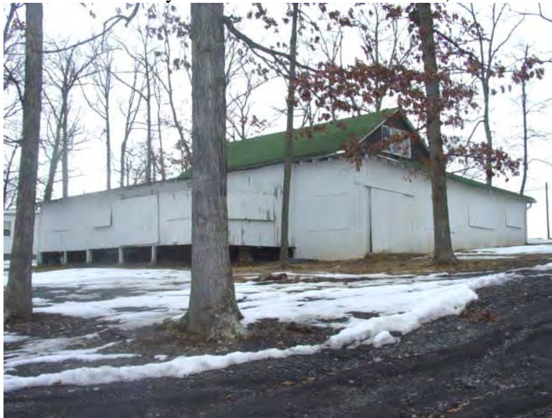
Figure V-11: The tabernacle at Damascus, at the core near the top of the open U, or horseshoe plan there. (Elizabeth Jo Lampl, Montgomery County Historic Preservation Section).
