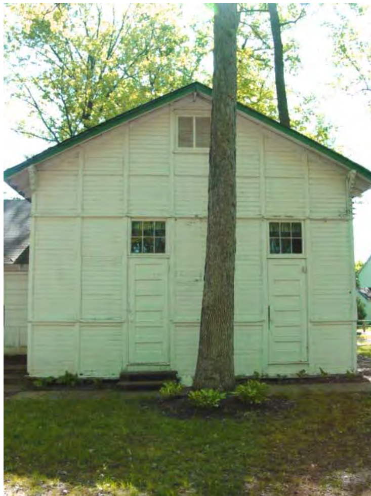
Figure VI-30: Portion of the dining hall at Spencerville Camp Meeting that was built as a World-War I era portable schoolhouse in Washington, D.C. (Elizabeth Jo Lampl, Montgomery County Historic Preservation Section)
