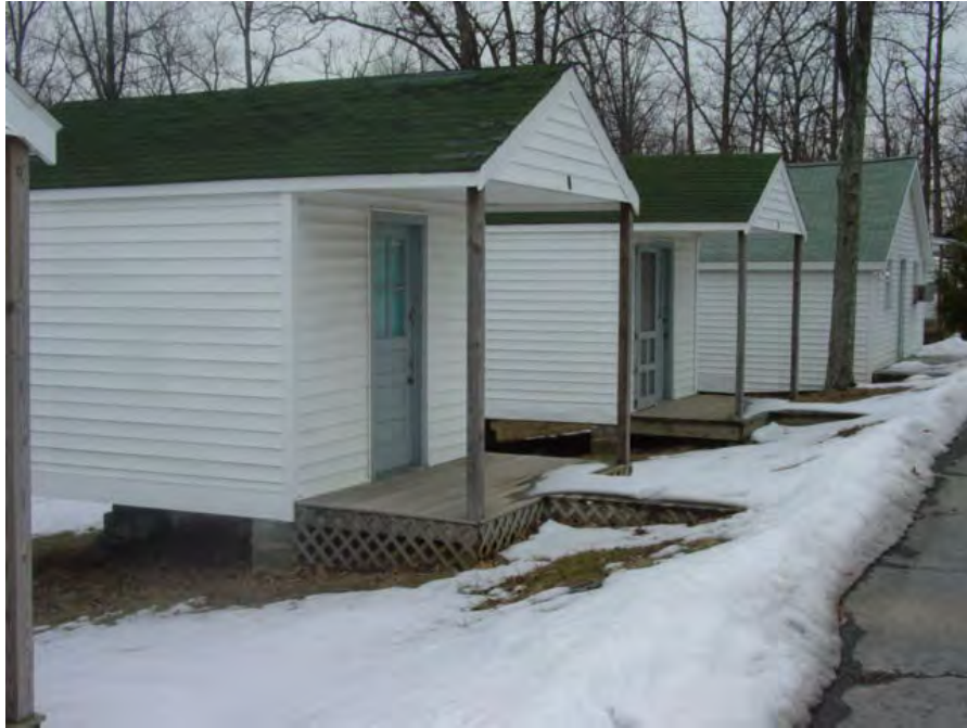
Figure VI-18: Damascus cottages re-sided in vinyl or aluminum, with new asphalt shingle roofs and new wood posts and decks. Several of the cottages have been maintained in this fashion. (Elizabeth Jo Lampl, Montgomery County Historic Preservation Section)
