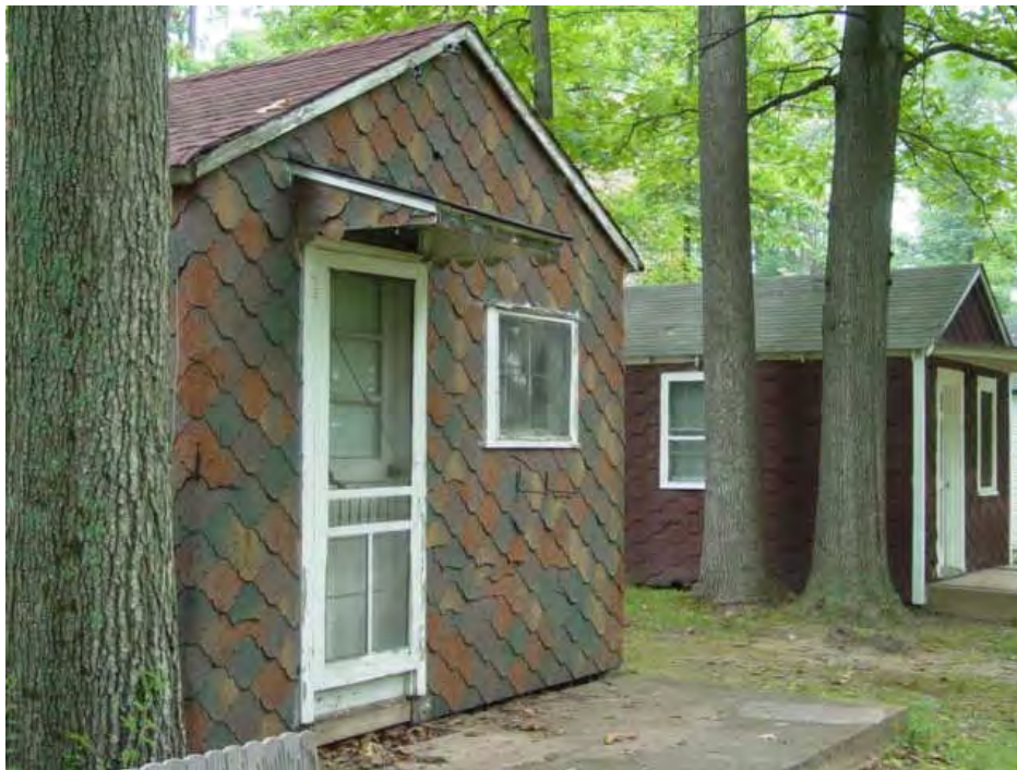
Figure VI-13: Asphalt shingle cottages that could date from the 1930s to the 1950s at Spencerville. (Elizabeth Jo Lampl, Montgomery County Historic Preservation Section)
