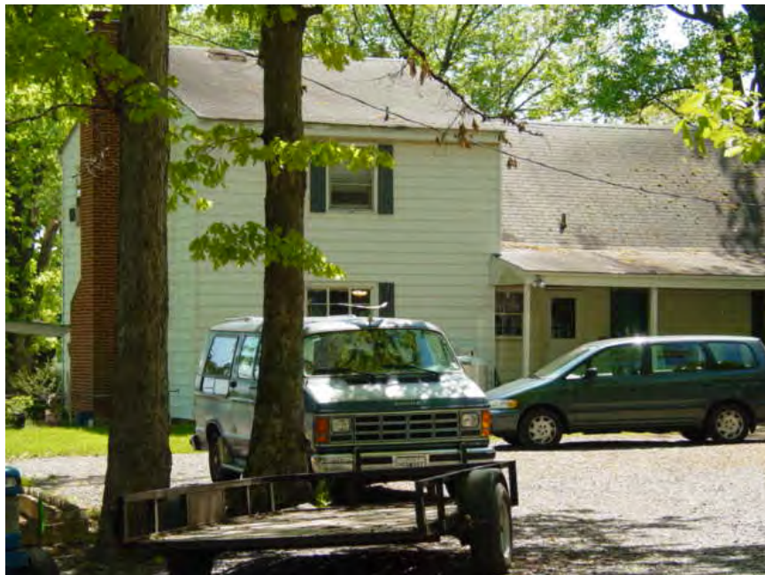
Figure VI-42: The groundskeeper's cottage at Spencerville. The Cape cod section at the right is the older section. (Elizabeth Jo Lampl, Montgomery County Historic Preservation Section)
