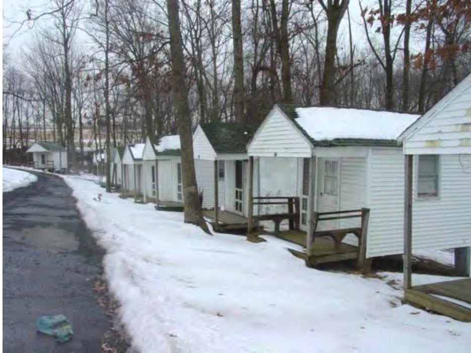
Figure IV-44: View of cabins and interior horseshoe road that winds through campground. (Elizabeth Jo Lampl, Montgomery County Historic Preservation Section)
