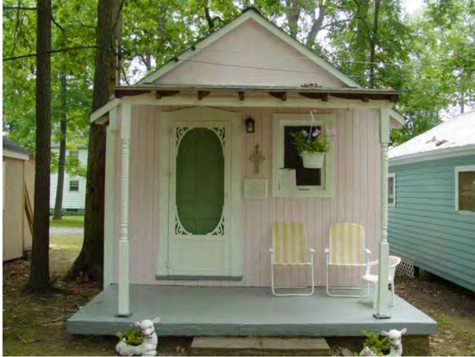
Figure VI-12: A ‘restored’ cottage in Spencerville, which is now well maintained, thanks to a pair of hardworking individuals. The original beadboard has been overlaid with T-111, and the unadorned wood posts have been replaced with the jigsawn type. The Victorian-style screened door is new. (Elizabeth Jo Lampl, Montgomery County Historic Preservation Section)
