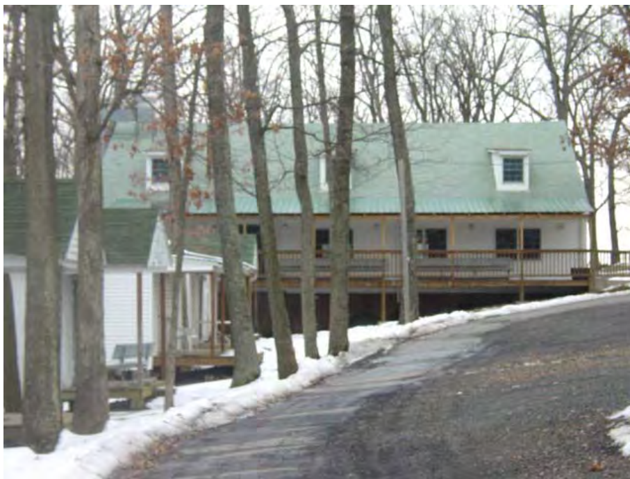
Figure V-2: Trees both line the perimeter road and are found behind the cottages at the Damascus Camp Meeting. (Elizabeth Jo Lampl, Montgomery County Historic Preservation Section)
