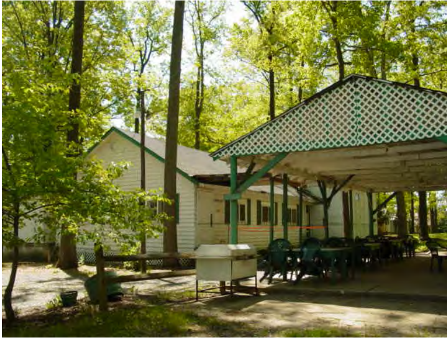
Figure VI-33: The dining hall/kitchen and adjacent, open-air picnic area at the Spencerville Camp Meeting. (Elizabeth Jo Lampl, Montgomery County Historic Preservation Section)
