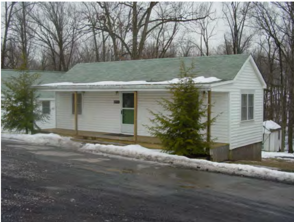
Figure VI-44: The office, one of the public service buildings at Damascus Camp Meeting. (Elizabeth Jo Lampl, Montgomery County Historic Preservation Section)
