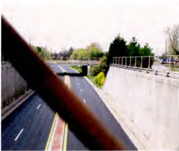
Figure 13: US 50 looking west towards Baptist Street, Salisbury (photo by Carol Ebright, SHA, 2007)
