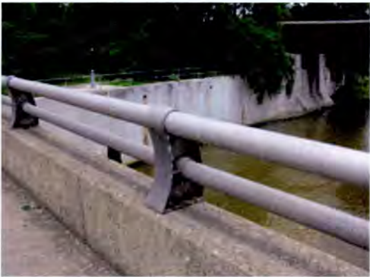
Two-strand aluminum railing and concrete parapet
