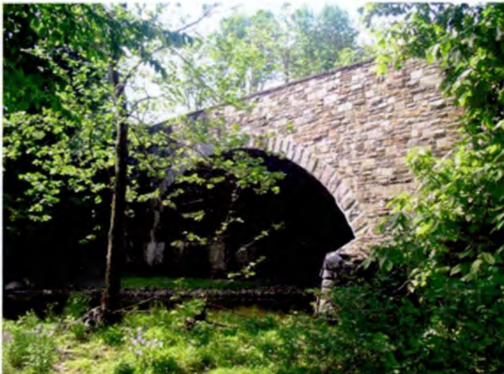
Figure 2: US 40 over Middle Creek, Frederick County (Photograph by John Hudacek, KCI, 2007)
