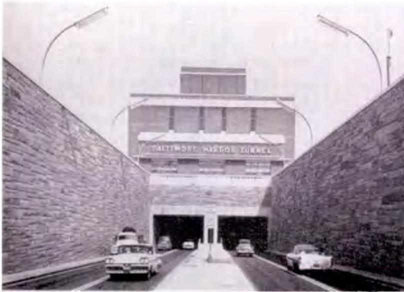
Figure 11: Baltimore Harbor Tunnel Entrance, 1958
