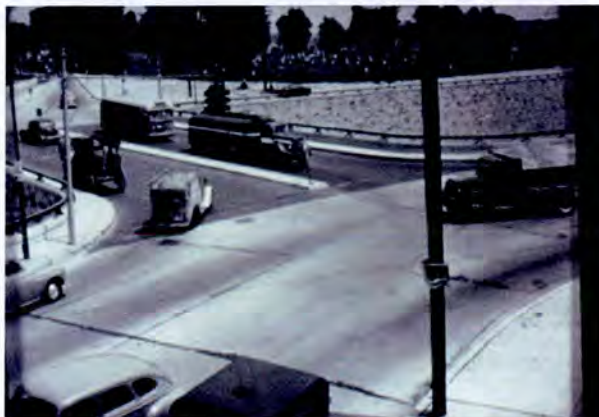
Figure 8: Water Street over MD 295 Interchange (Source: SHA Photo Archive)
