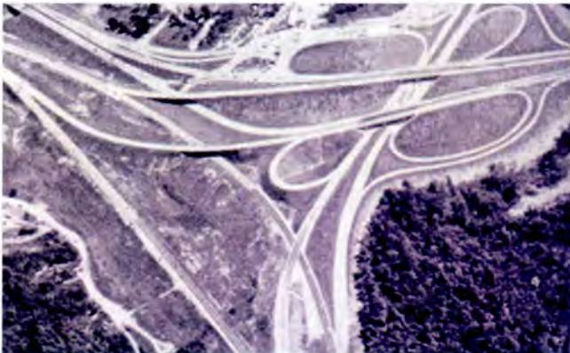
Figure 5: MD 295 and MD 201 and US 50 Interchange, Prince George's County. One "paperclip ramp" is in the northwest corner of the interchange. 36
