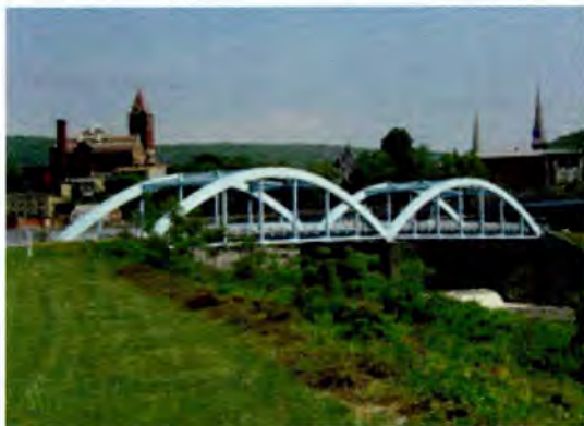
Steel Through Arch (SHA Bridge No. 0106600 -- Blue Bridge, Cumberland, MD)
