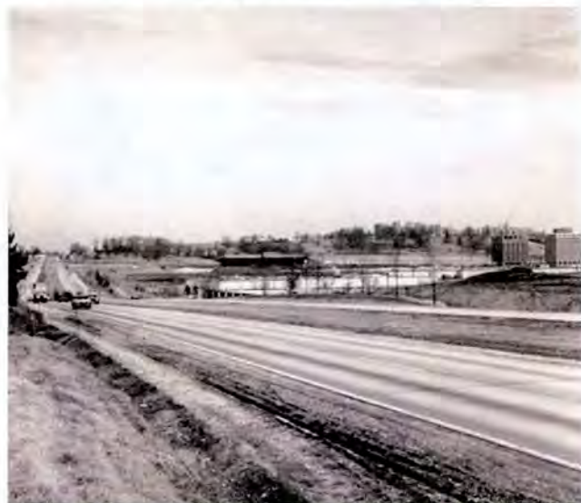
Figure 15: I-83 looking north towards Shawan Road (Source: SHA Photo Archive)
