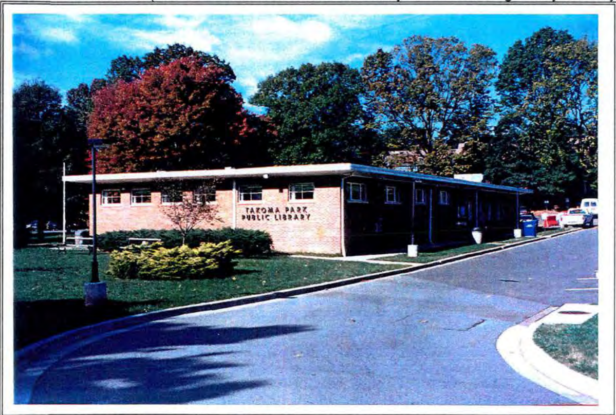
Plate 33: Library (Maple Avenue, Takoma Park, Montgomery County)
