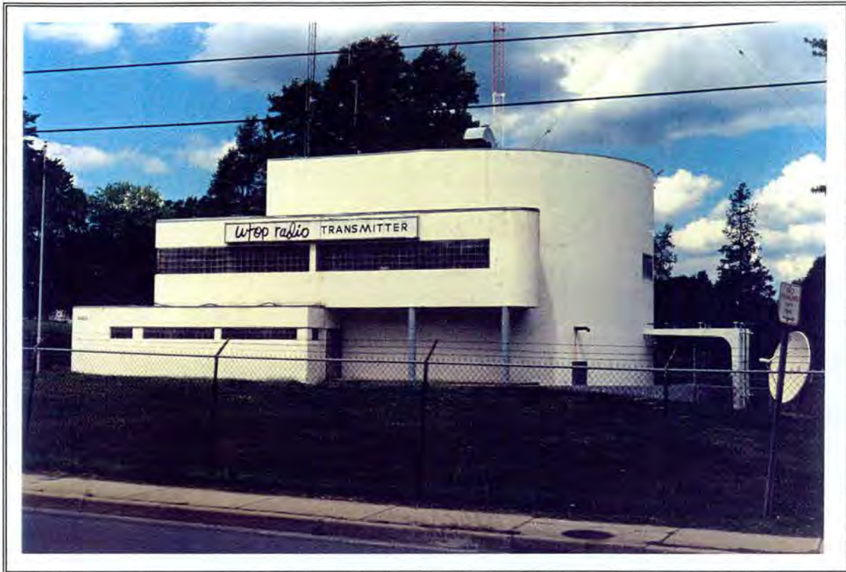
Plate 2: "Streamlined" building (WTOP Radio, 2021 University Blvd., Wheaton)
