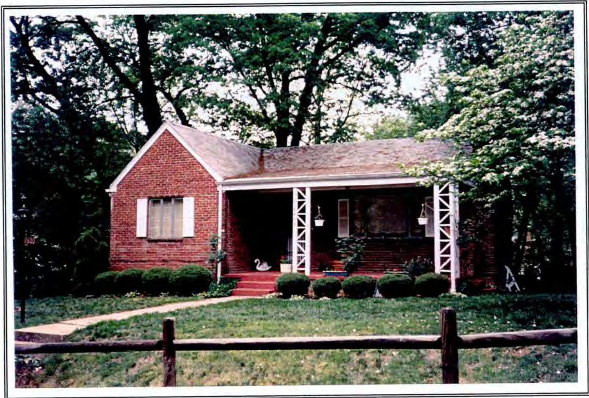
Plate 19: Minimal Traditional House (9800 Grayson Avenue, Four Corners, Montgomery County)
