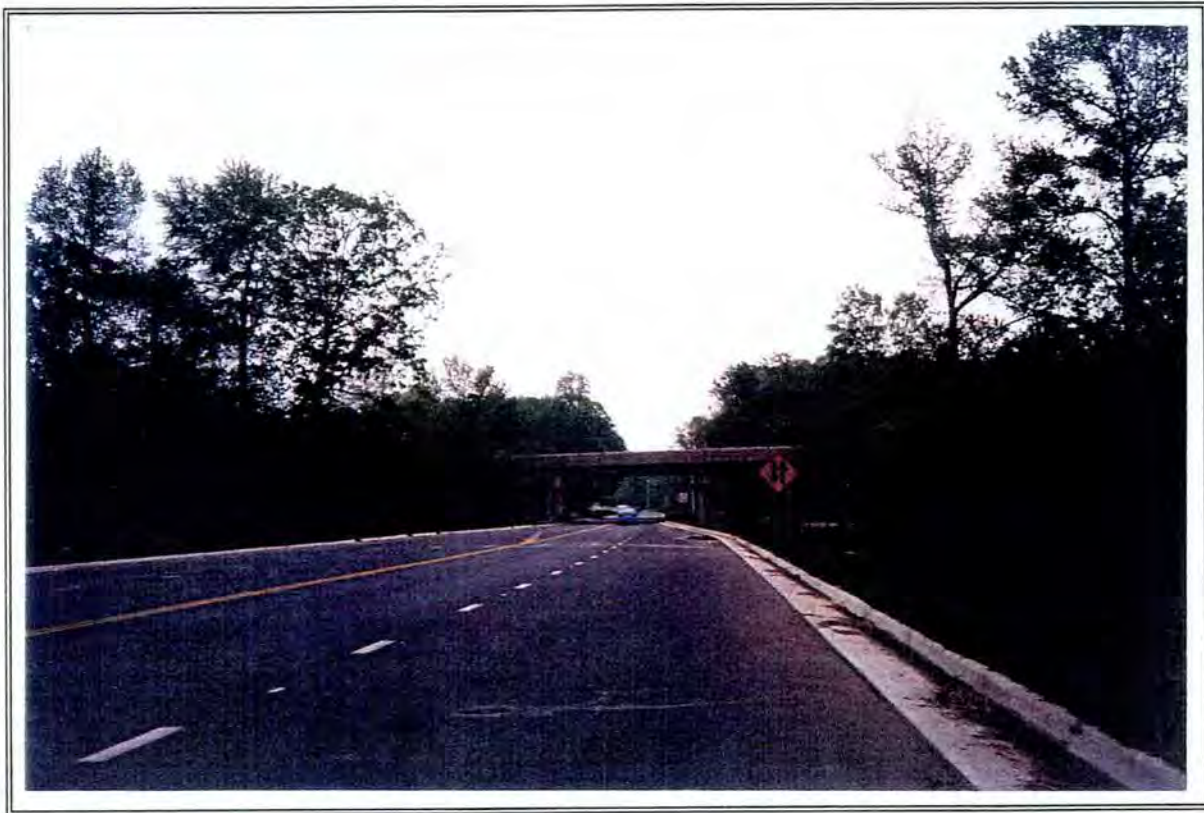
Plate 42: Parkway (Suitland Parkway at Capital Beltway (I-495), Prince George's County)
