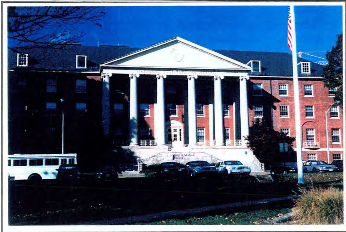
Plate 38: Hospitals (National Institutes of Health, Building #1, Bethesda, Montgomery County)
