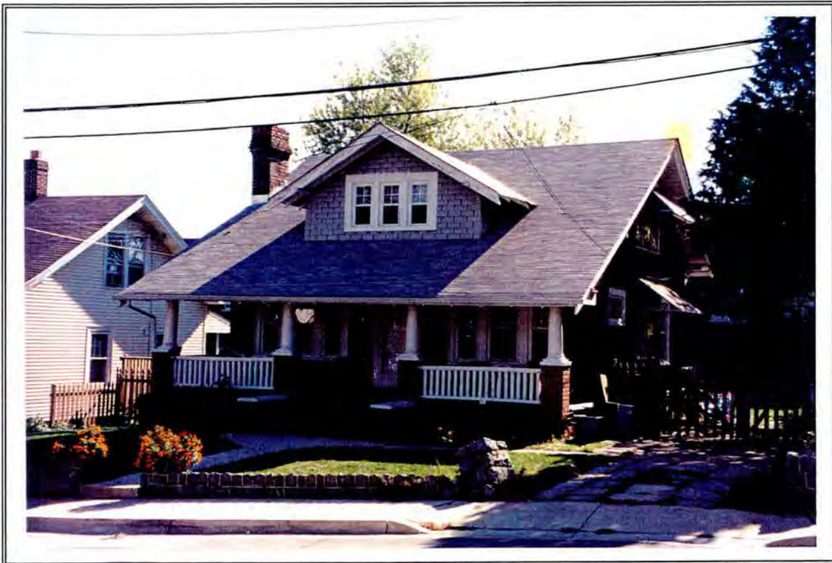
Plate 15: Bungalow (4400 block of Gallatin Street, Hyattsville, Prince George's County)
