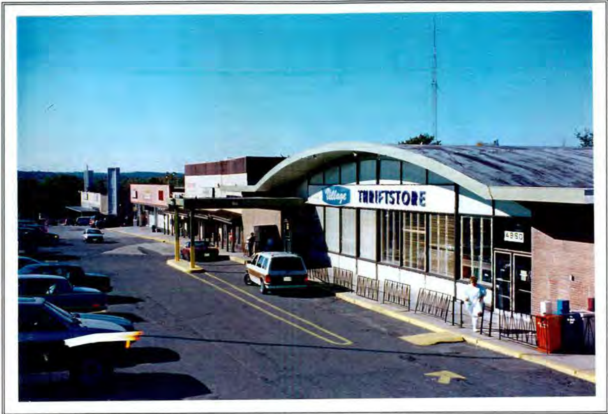
Plate 3: Standard shopping center (Village Thrift Shopping Center, 5600 Annapolis Blvd., Bladensburg)
