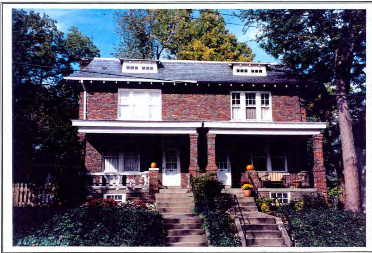
Plate 21: Double House/Duplex (3637-3639 Jenifer Street, Washington, D.C.)
