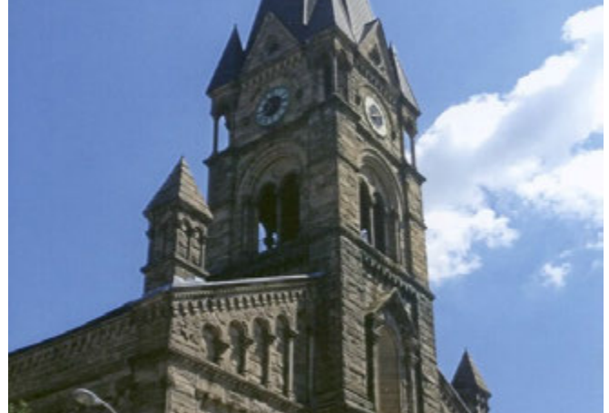
St. Michael's Church Complex
