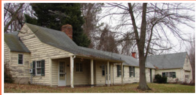
Gardener's Cottage prior to rehabilitation.
