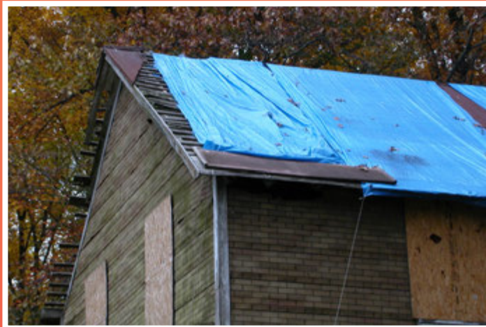
The lodge in 2007 prior to stabilization.
