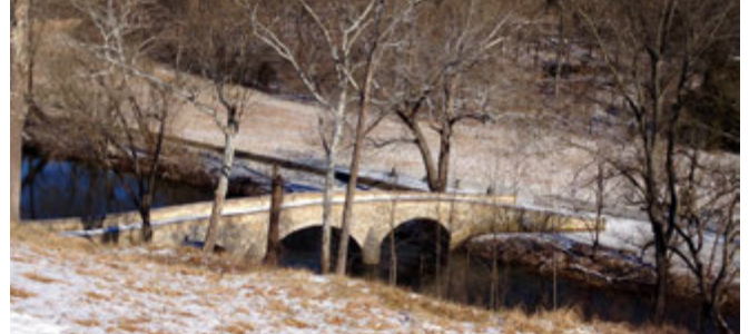
Antietam Burnside Bridge
