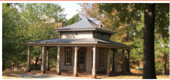
Watchbox at the Naval Support Facility Indian Head
