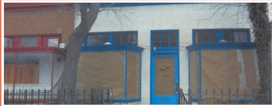
The Harvey Dairy Store before rehabilitation.
