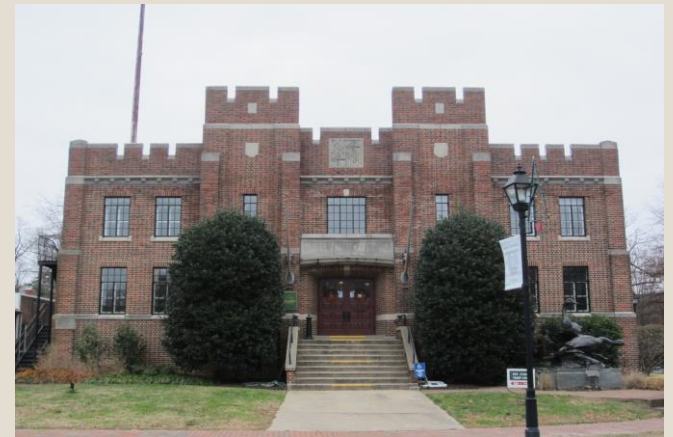
Easton Armory, Talbot County
