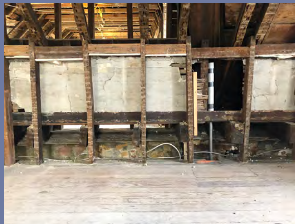
The original floor level and plaster wall sitting about two feet above the existing floor. Note the black-painted baseboard and pieces of the intact plaster wall above.
