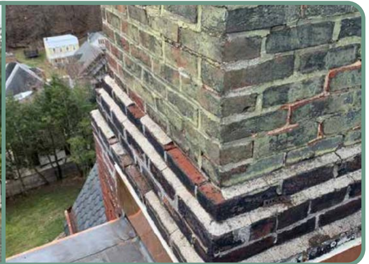
FY24 homeowner project to fix chimney flashing
