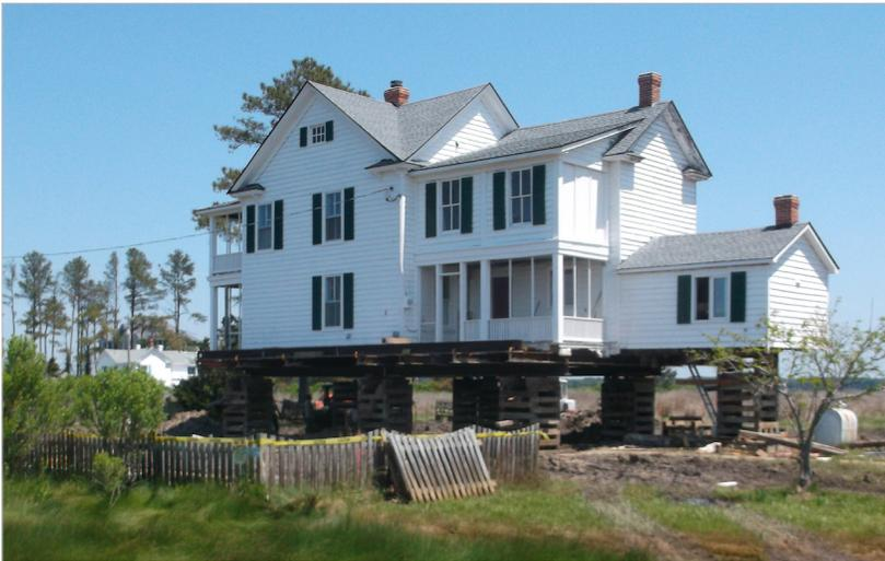
Figure 2.38- Elevation in progress of a late-19th century historic home on St. George Island, St. Mary's County. The building was elevated to the BFE plus three feet of freeboard. (Source: MEMA)
