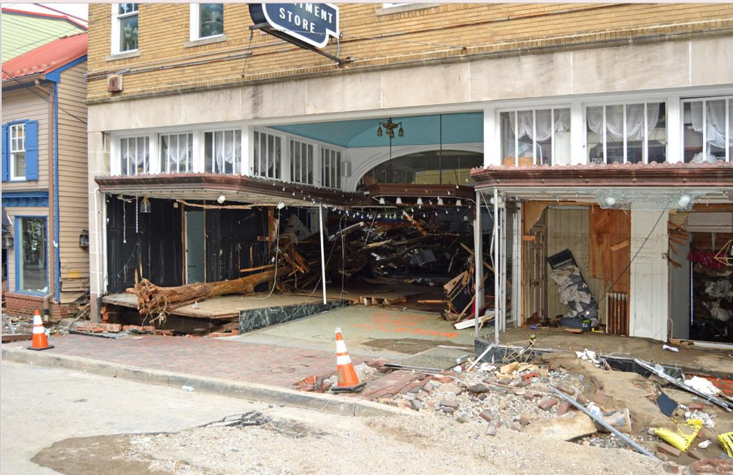
*Figure 2.23 - A tree was found lodged in the storefront during initial damage assessments after the 2016 flash flood in Ellicott City. Although the storefront glazing system was lost, its cornice and the transom windows above can be stabilized and retained in the rebuilding process.*
