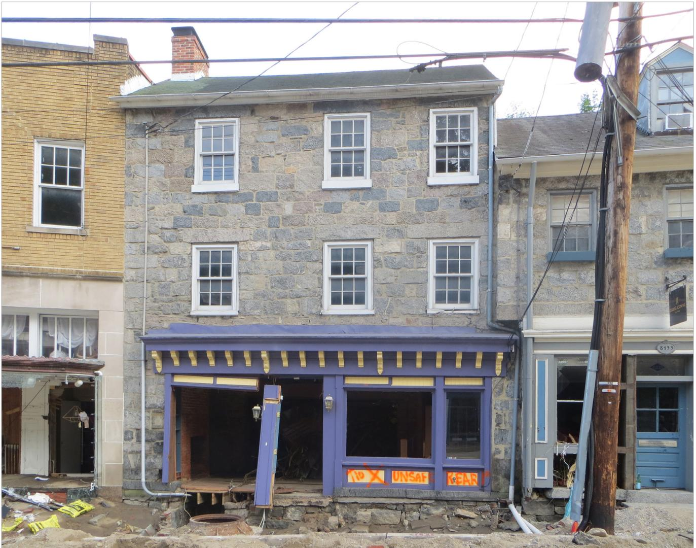
Figure 2.21 - Building Tagged as "Unsafe Rear" by an assessment team. The rear wall of the first floor was blown out due to floodwater entering the front of the building. Ellicott City, Howard County, 2016.
