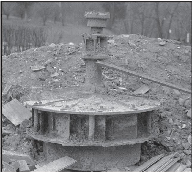
Figure 11: Pierce Mill, Washington, D.C., water turbine (Courtesy of the National Park Service, date unknown).
