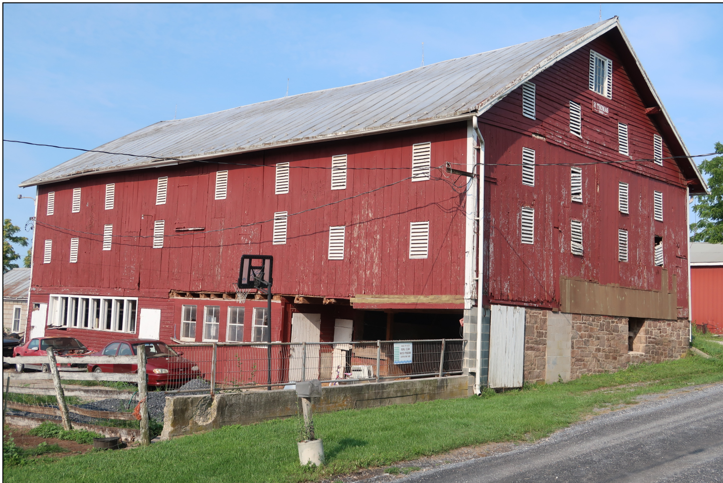
Figure 11. Example of bank barn from the Thomas Farm in Keymar, Maryland that was converted in the twentieth century for dairying. On the lower level of the barn the once over-hanging forebay has been enclosed.
