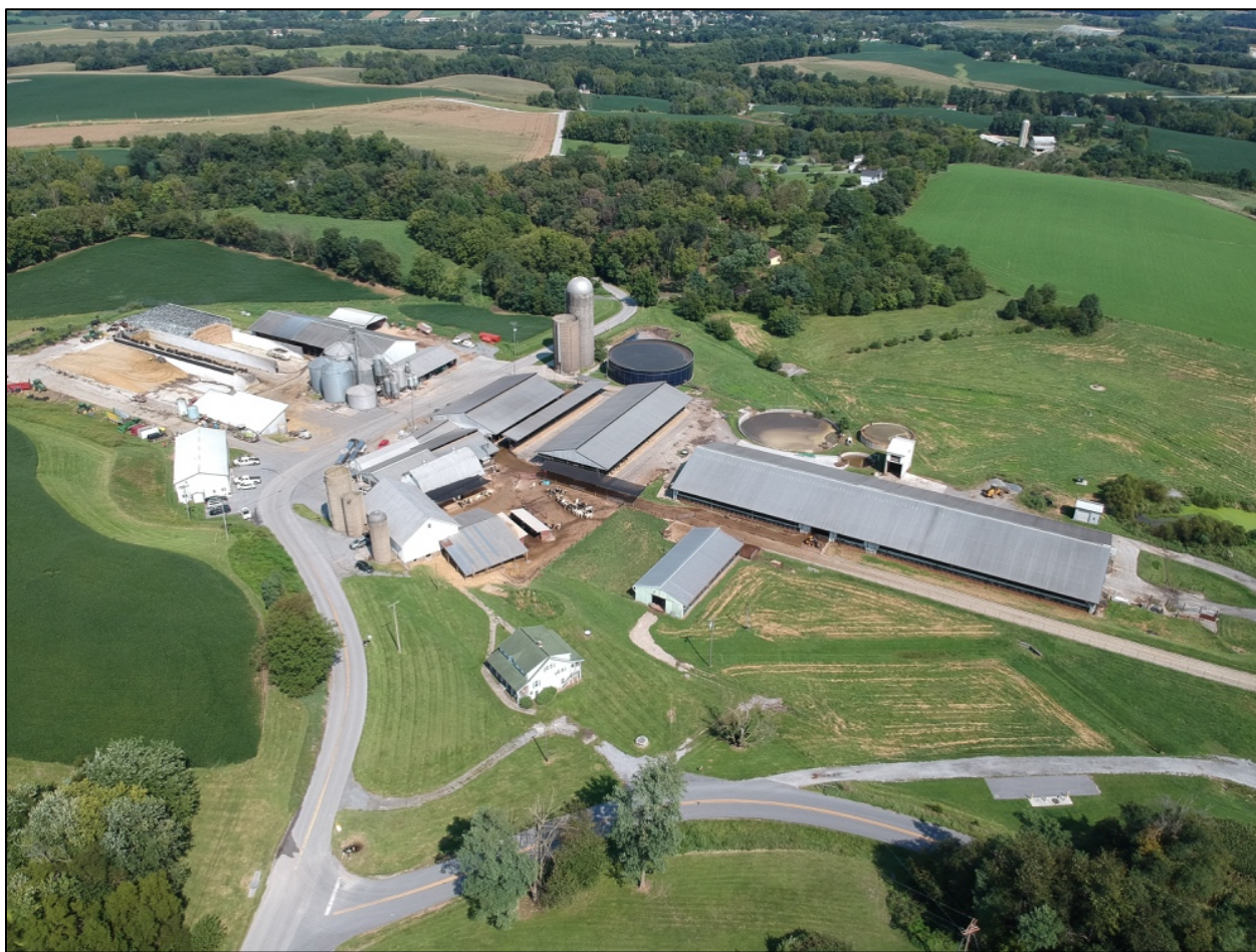
Figure 15. Aerial view showing the Coldsprings Farm showing the center of the dairy complex, looking northeast (Michael J. Emmons, Jr. 2021).
