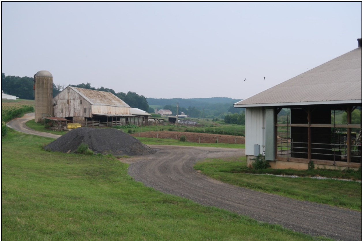
Figure 19. Environmental view of the P. Peterman Farm, showing the bank barn in the background and a modern heifer barn in the foreground, looking northwest (Michael J. Emmons, Jr., 2021).
