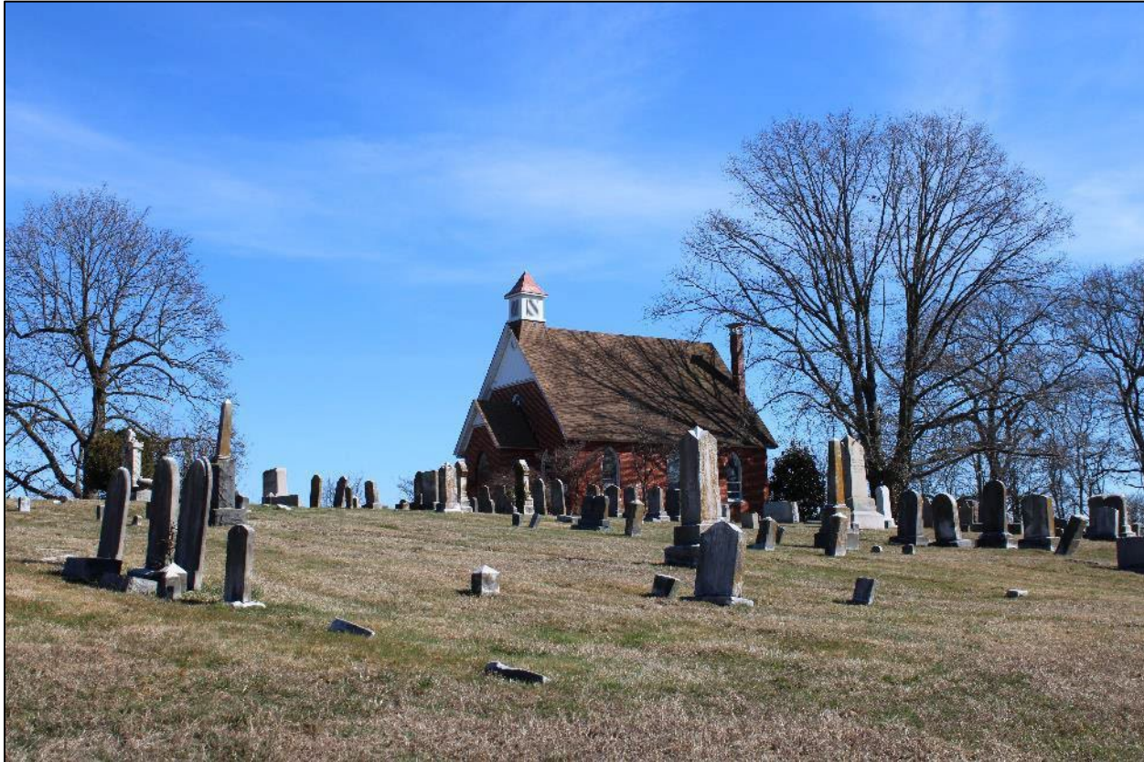
Figure 17: Photo of Cokesbury Methodist Church in Abingdon. EHT Tracerics (March 2024).
