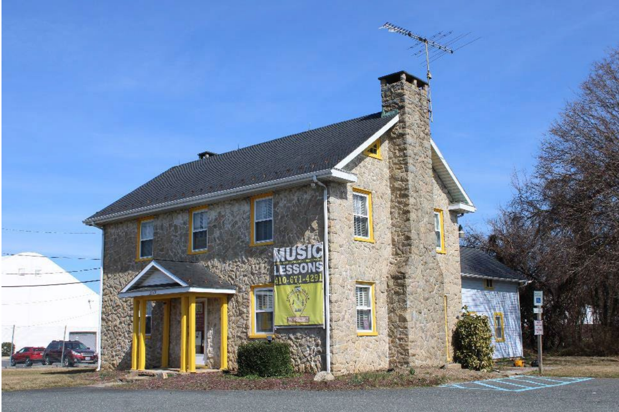
Figure 20: The Peery Stone House (M: HA-2301), East and South Elevations, Looking North
