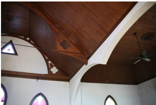
Figure 43, Asbury M. E. Church, interior, decorated roof trusses with iron tie rods, Paul B. Touart, photographer, 2.2018.
