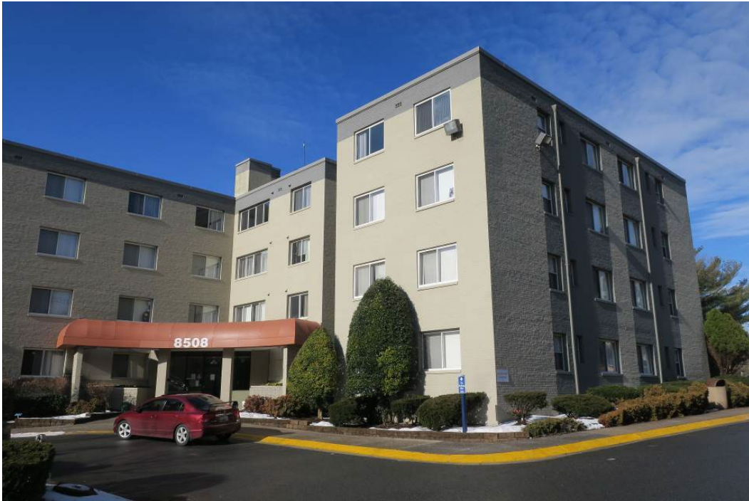
Figure 6: Summit Hill Apartments, 8508 16 th Street, looking west
