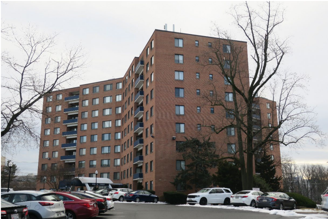
Figure 7: Summit Hill Apartments, 8484 16 th Street (the y-plan nine-story apartment building, looking east)
