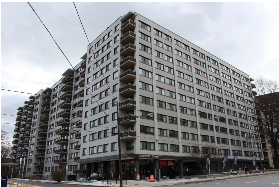
Figure 8: Colesville Tower, looking southeast
