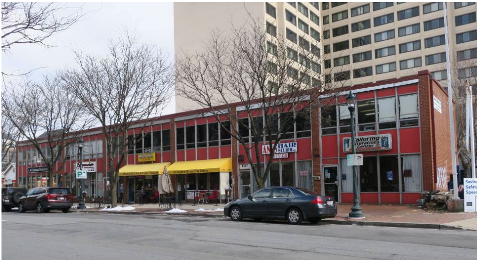
Figure 30: Montgomery Realty Building, West elevation, looking northeast.
