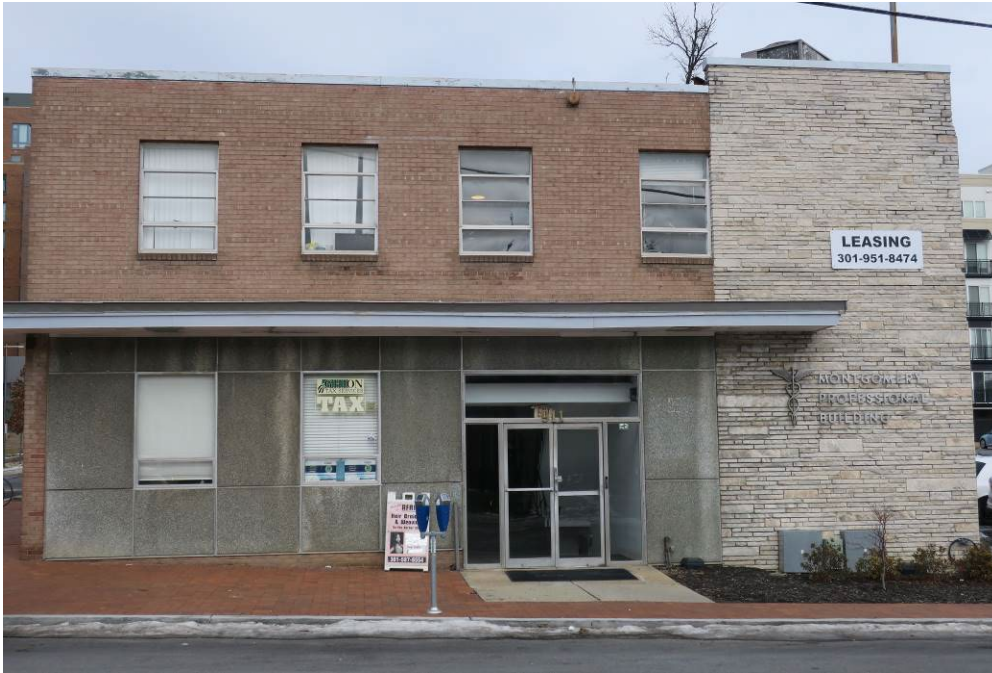
Figure 32: Montgomery Professional Building, South elevation, looking north.
