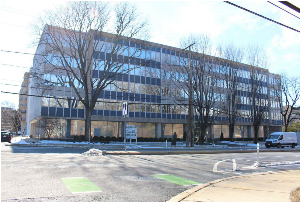
Figure 27: Operational Research Inc. Building, North elevation, looking south.
