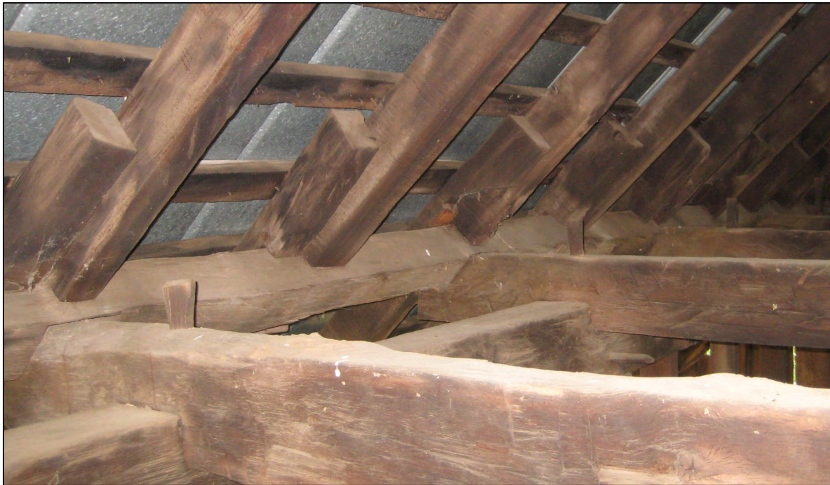
Figure 8. Even though the De la Brooke barn was originally outfitted with nailers to mount rows of wood shingles, the rafters were set in the traditional close-spacing of 2' that was suited to attaching clapboards.
