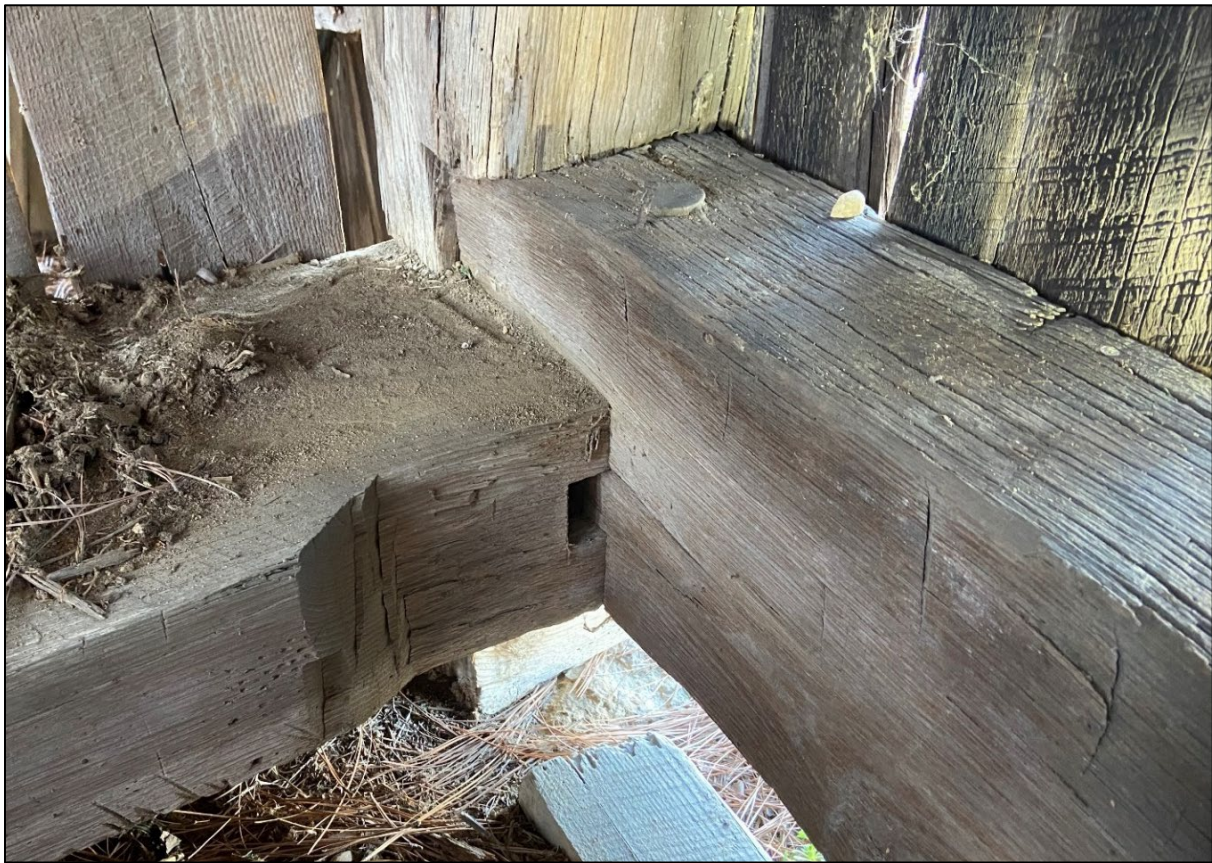
Figure 19. Buckler barn (CT-1090), double-tenoned corner joint with clenched post.
