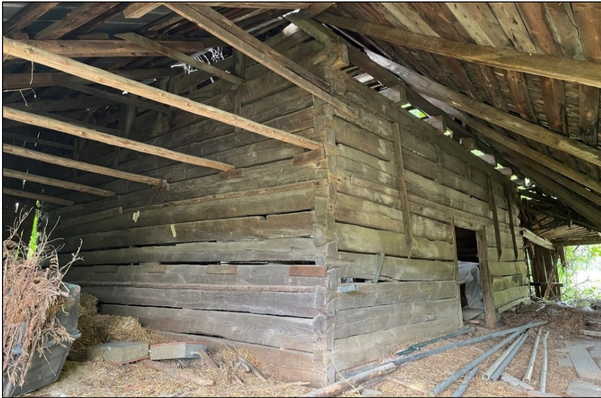
Figure 12. Spalding tobacco barn (SM-170). The well executed full-dovetail notching at the corners testifies to the high level of skill of the builders, but also produced a relatively tight fit for the logs that is surprising given the need for ventilation to help cure the tobacco (facing northwest).
