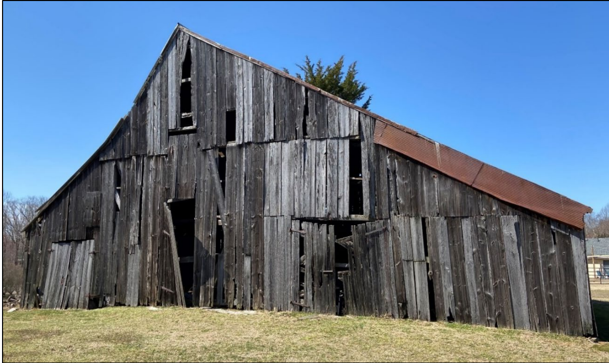
Figure 3. Buckler tobacco barn (CT-1090), with one original shed on the left and one added shed on the right; the barn is in fair condition with medium integrity (facing west).
