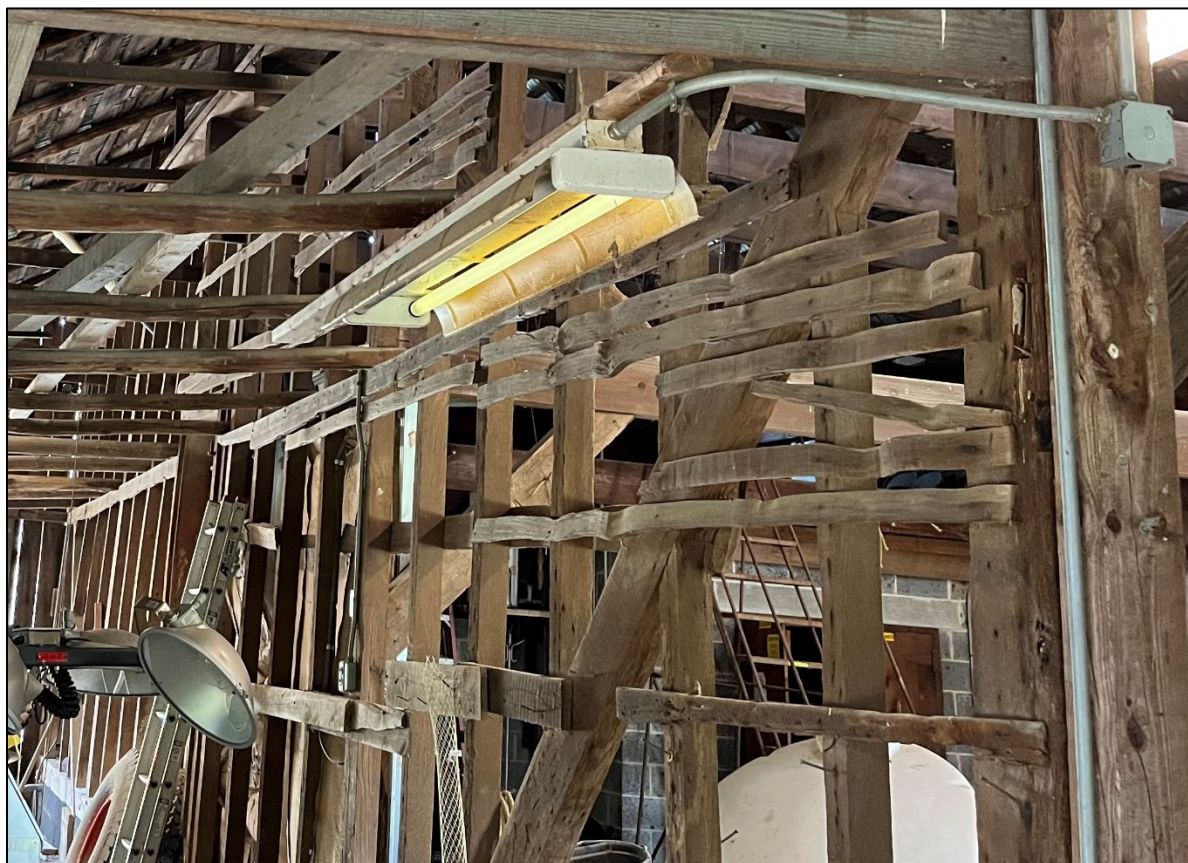
Figure 18. Parrans tobacco barn (CT-58) with remnants of a covering of spaced riven battens attached to the exterior wall facing the open-sided shed.
