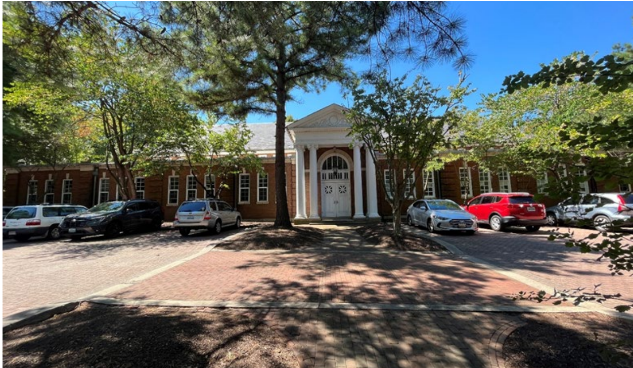
Figure 52: Northeast elevation of Iglehart Hall, looking southwest. EHT Traceries, August 2023.
