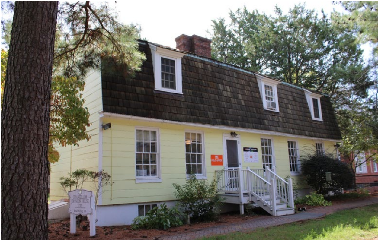
Figure 47: Northwest elevation of the Johnson House, looking south. EHT Tracerics, October 2023.
