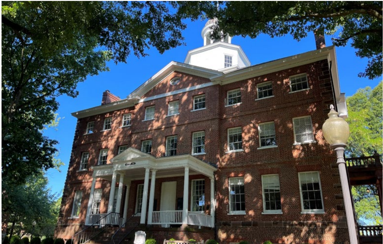
Figure 44: East elevation of McDowell Hall, looking west. EHT Tracerics, August 2023.
