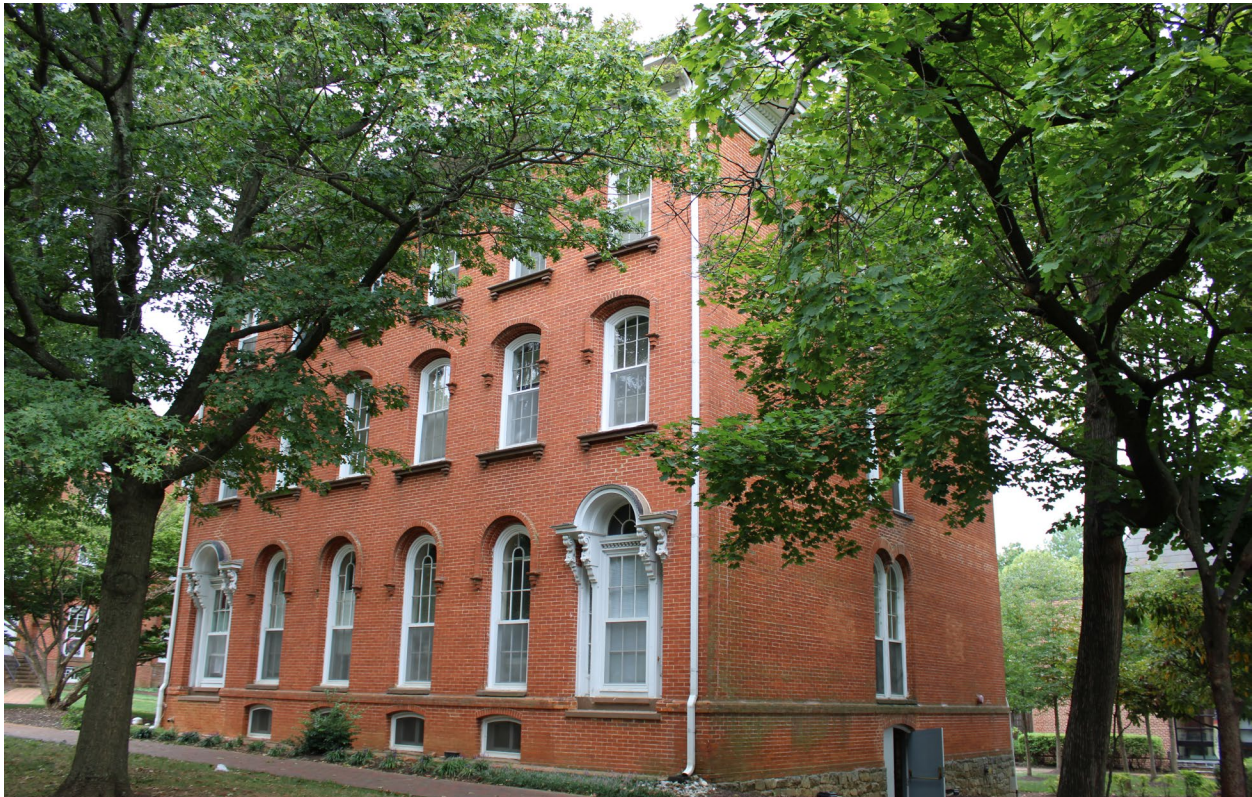
Figure 41: Northwest elevation of the Chase-Stone House, looking southeast. EHT Tracerics, August 2023.
