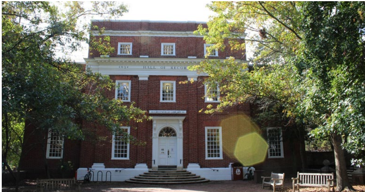
Figure 50: Northeast elevation of the Maryland Hall of Records, looking southwest. EHT Traceries, October 2023.
