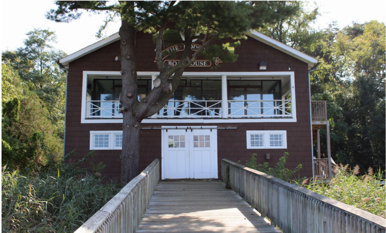
Figure 53: Northwest elevation of the Beneficial-Hodson Boathouse, looking southeast. EHT Tracerics, October 2023.
