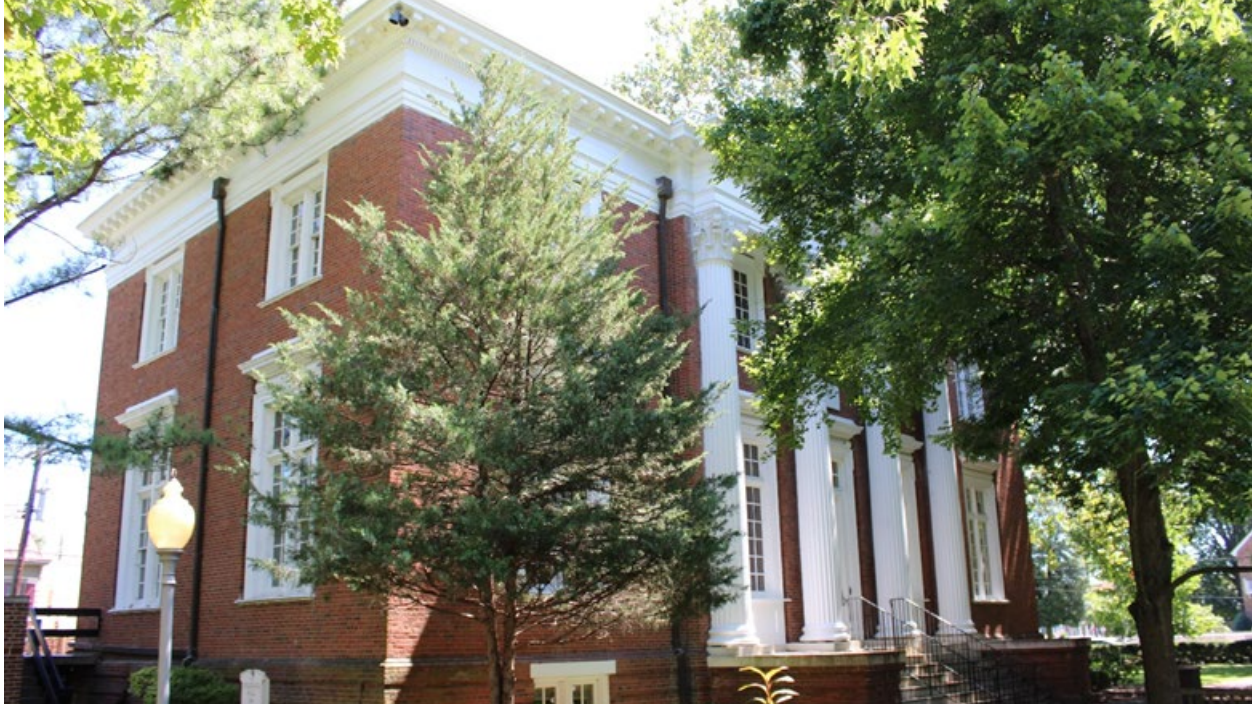
Figure 42: Southwest (front) and northwest elevations, looking east. EHT Tracerics, August 2023.
