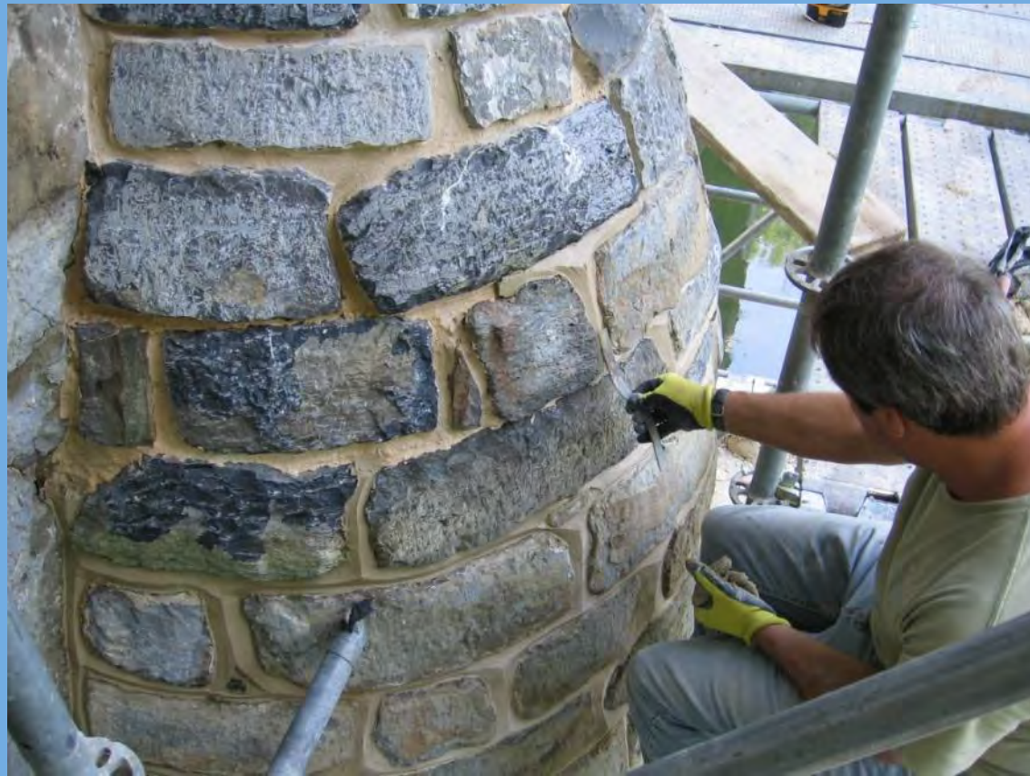
Repointing masonry on Conococheague Stone Arch Bridge in Williamsport
