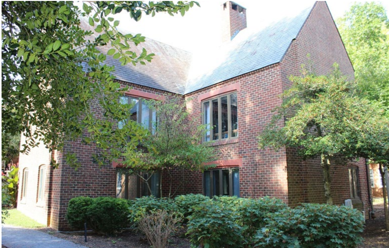
Figure 56: East corner of the Harrison Alumni Center, looking southwest. EHT Traceries , October 2023.
