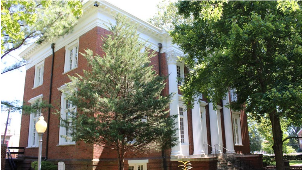
Figure 42: Southwest (front) and northwest elevations, looking east. EHT Tracerics, August 2023.
