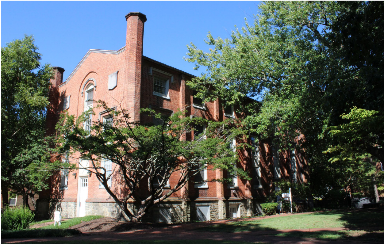
Figure 45: Southwest elevation of Humphreys Hall, looking northeast. EHT Tracerics, August 2023.
