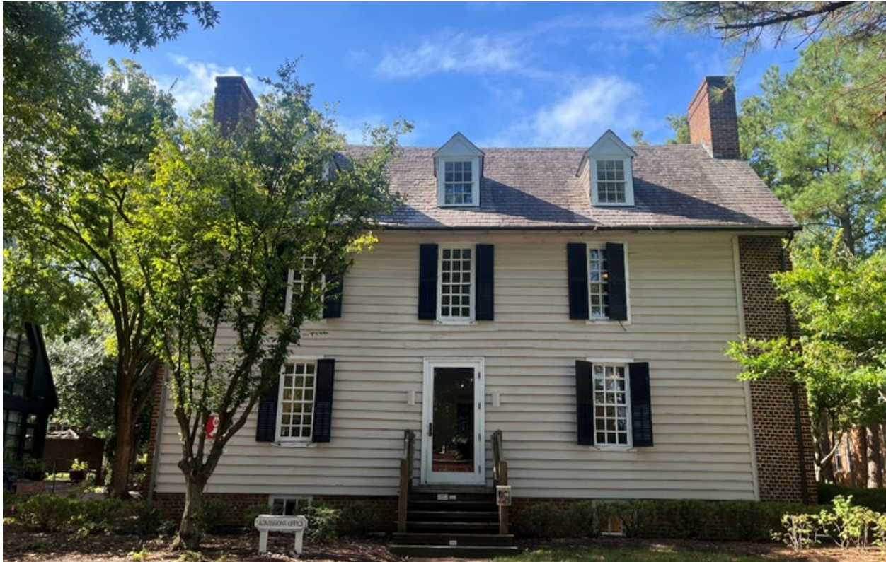
Figure 40: Northwest elevation of the Charles Carroll the Barrister House, looking southwest. EHT Tracerics , October 2023.
