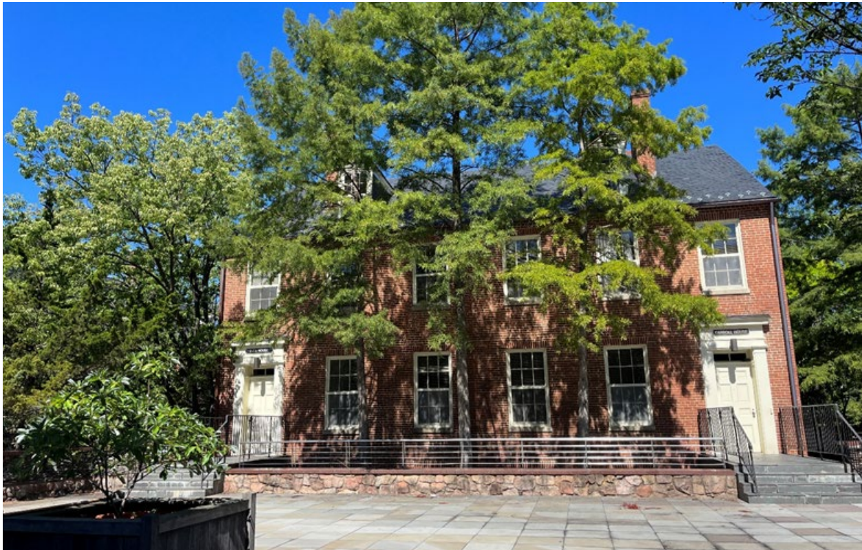
Figure 46: Southeast elevation of Paca-Carroll House, looking northwest. EHT Tracerics, August 2023.
