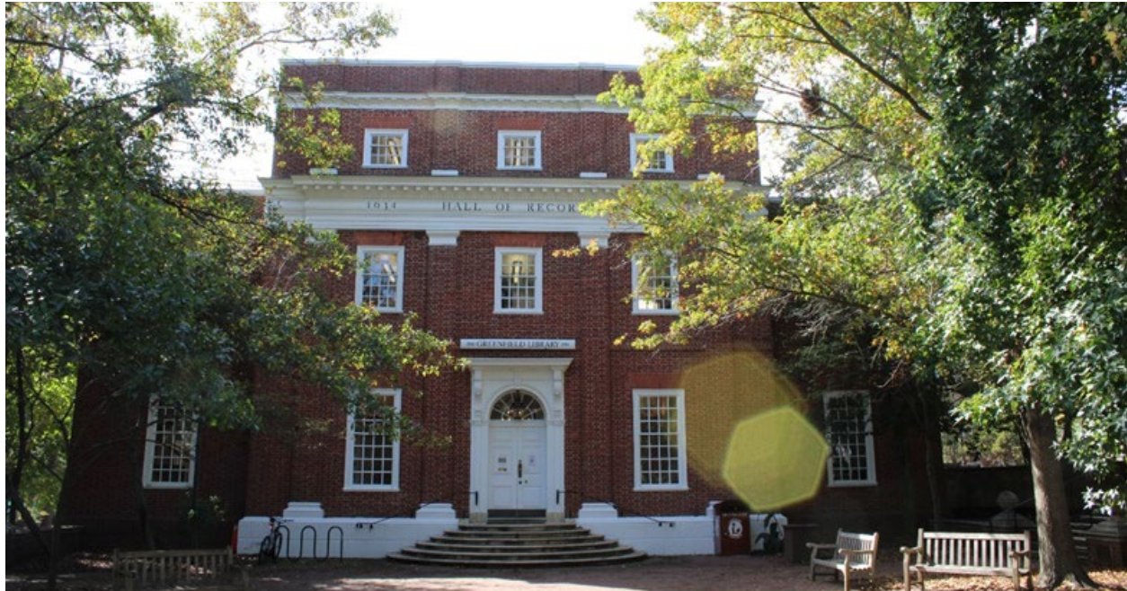
Figure 50: Northeast elevation of the Maryland Hall of Records, looking southwest. EHT Traceries, October 2023.
