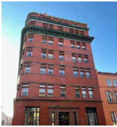
Liberty Trust Bank Building – Allegany County ($1.5 million) Cumberland architect Wright Butler designed the six-story Liberty Trust Bank Building, built in 1907, which reflects early 20th-century commercial growth in the region.
