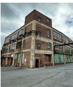
Building 51B/46C – Crown, Cork, and Seal Highlandtown Plant – Baltimore City ($2.1 million)
