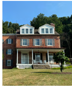
Holly Hill – Baltimore City ($320,000) Built c. 1801, this Federal-style house is among Cockeysville's oldest standing buildings, linked to the early milling, agriculture, and water-powered industries. Now located within the Broadmead retirement
