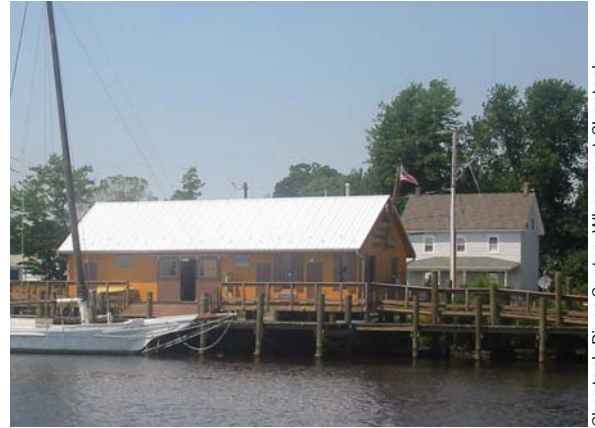
Choptank River Center, Wharves at Choptank Crossing, Denton, by Kate Wise
