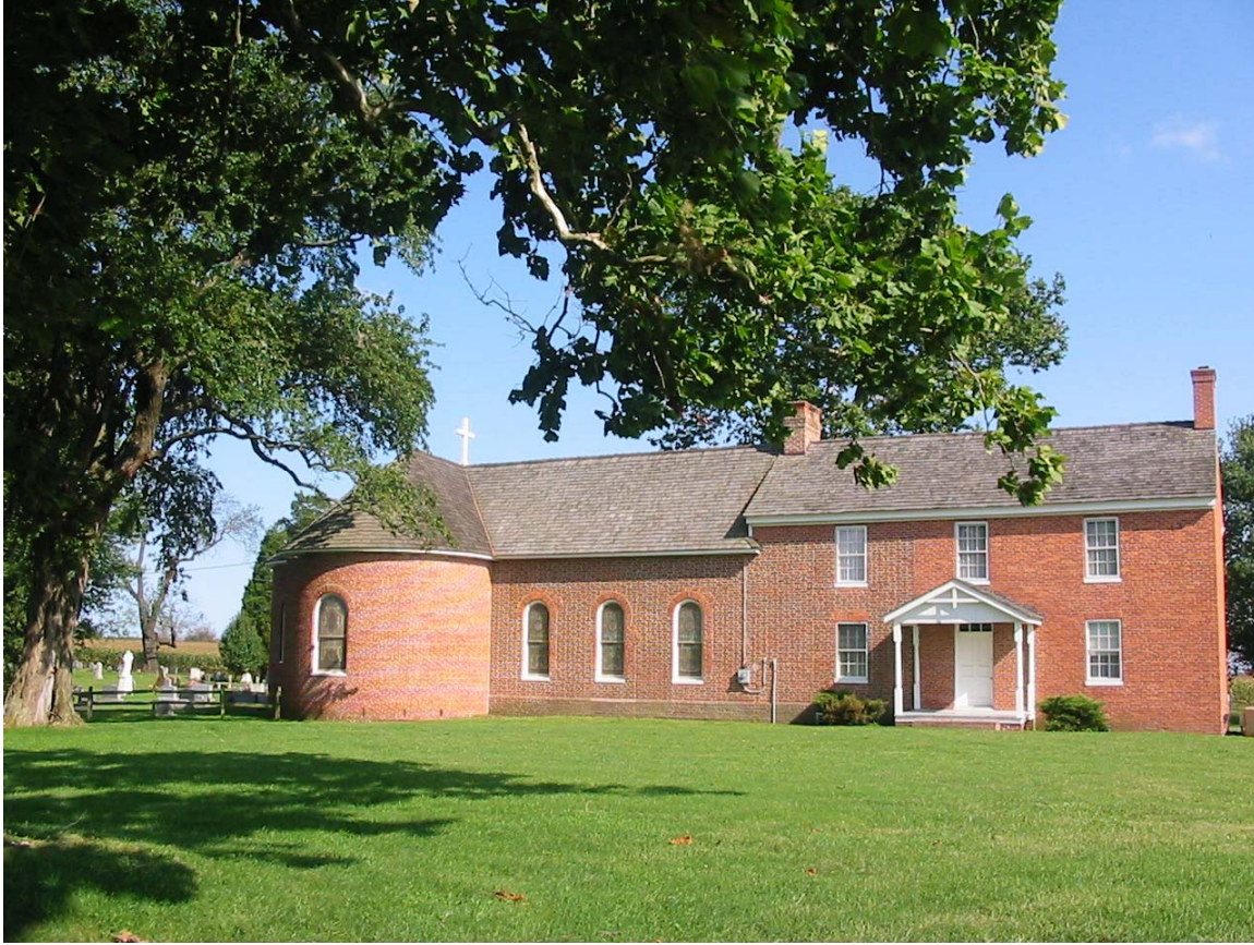
Figure 3-25 St. Joseph's Roman Catholic Church, northern Talbot County
