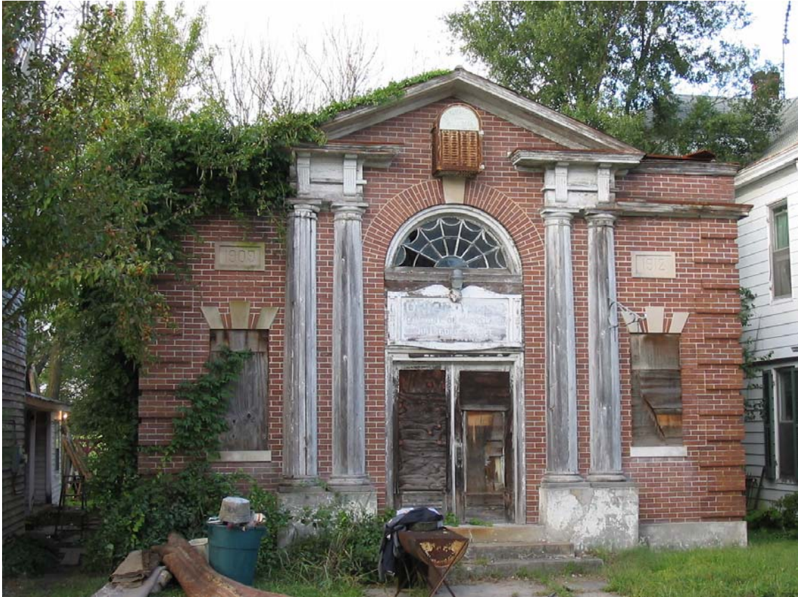
Figure 6-23 Old Hillsboro Bank and New Hillsboro Town Hall
