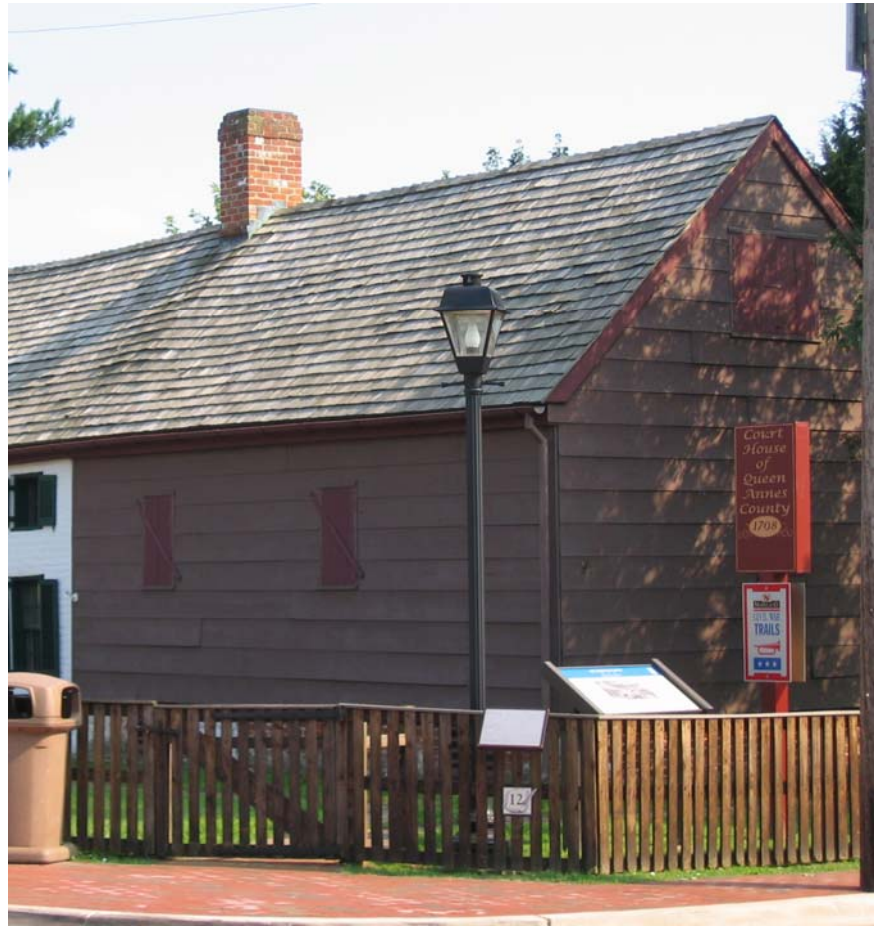
Figure 3-1 Old Queen Anne's County Courthouse, Queenstown
