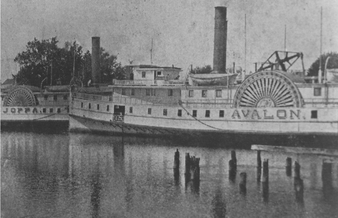
Figure 5-10 Avalon Floating Theatre
