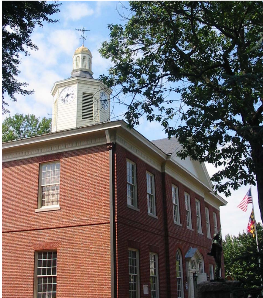
Figure 8-2 Talbot County Courthouse, Easton
