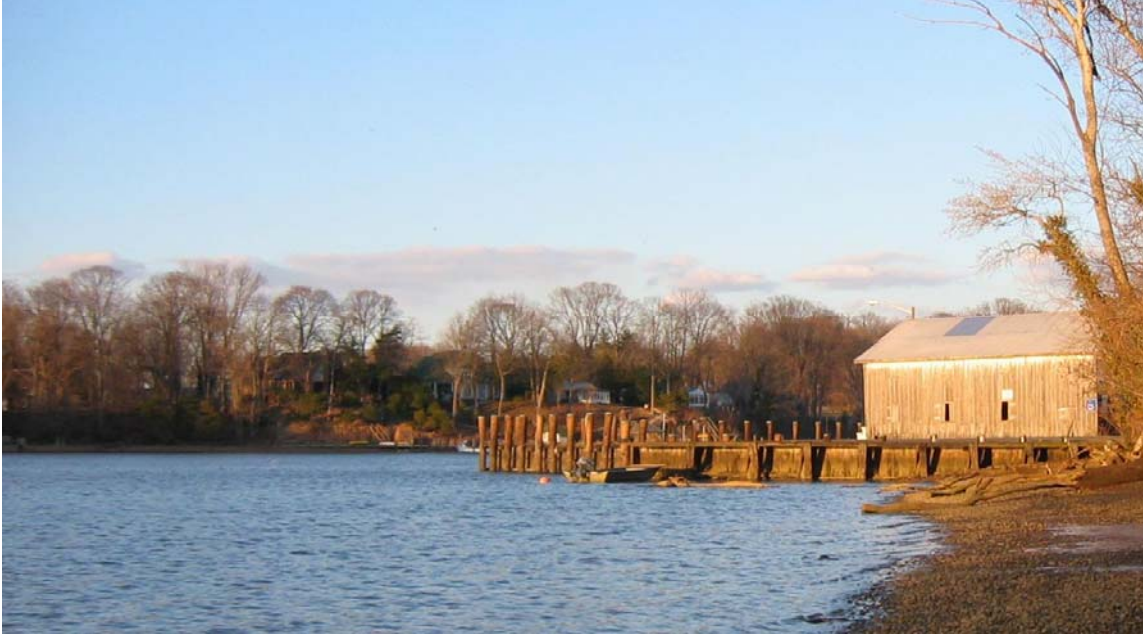
Figure 4-8 Turner's Wharf Granary
