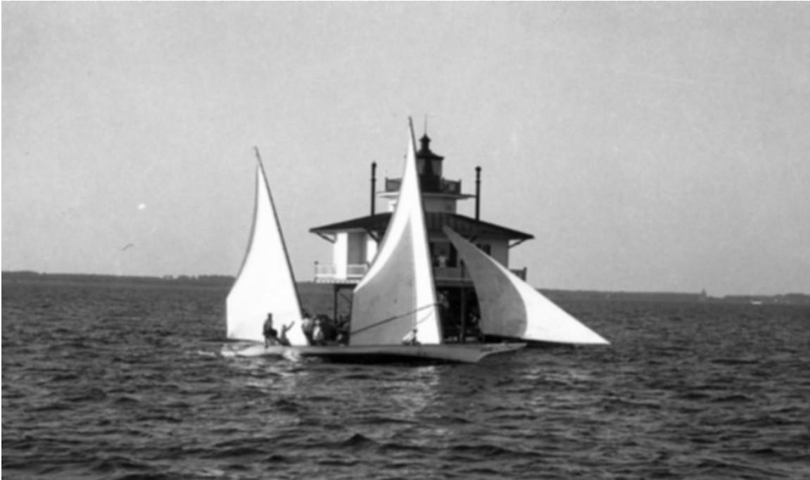
Figure 2-5 Log Canoe and Lighthouse (historic photo)
