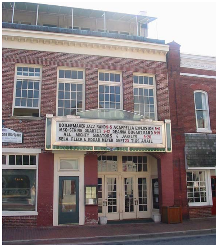
Figure 2-6 Avalon Theatre, Easton
