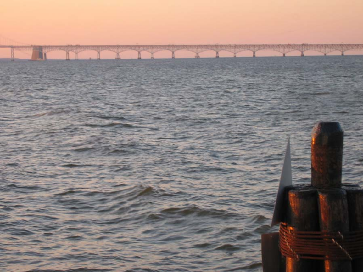
Figure 1-7 The Chesapeake Bay Bridge, seen from Matapeake Park, Kent Island “The Bay Bridge” is named for Governor William Preston Lane, Jr., who established the transportation authority that built the second span in 1973. The opening of the first span in 1952 inspired the founding of several historical societies in the region as residents realized their way of life was changing.
