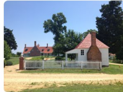
Sotterley Plantation gatehouse project. Photo provided by Nancy Easterling.
