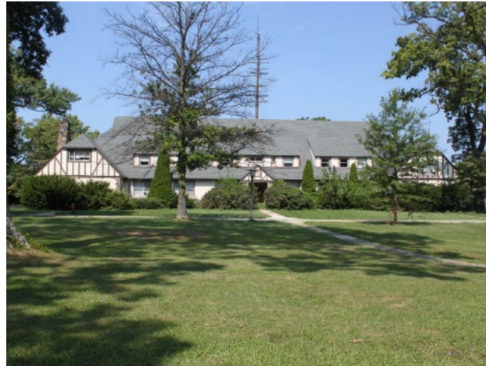
Figure 12: Pikesville Armory's Admin. Building 2 (Bernard D. Merson Building) . Courtesy of the Maryland Department of Planning – Maryland Historical Trust.
