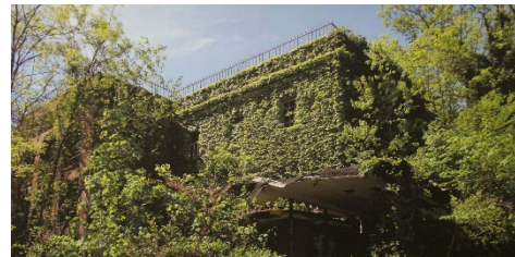
Figure 19: Exterior of a building on the campus of Glenn Dale Hospital, 2016. Courtesy of M-NCPPC.
