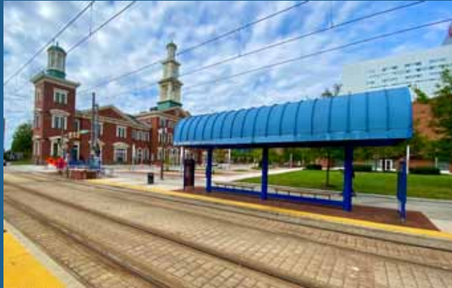
Historic Camden Station at MTA's Convention Center Light Rail stop in Baltimore City.
