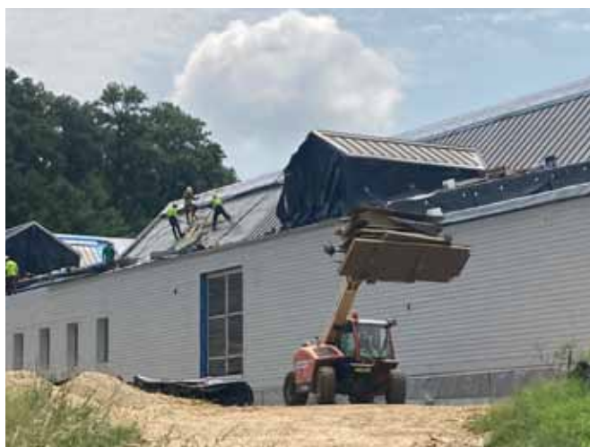
Left: MAC Lab roof replacement in progress.
