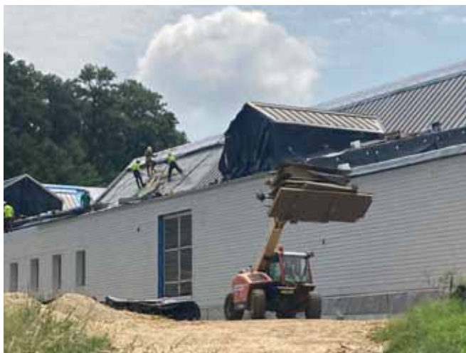
Left: MAC Lab roof replacement in progress.
