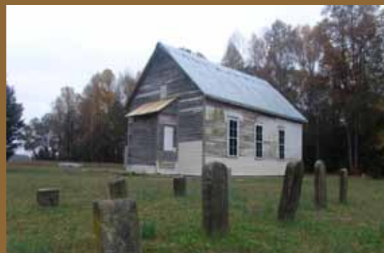
Bottom row: St. Paul Church after stabilization.
