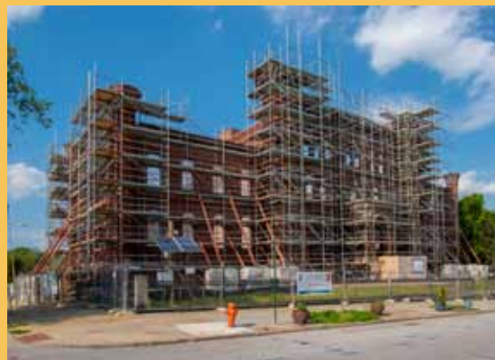
Above: After rehabilitation
