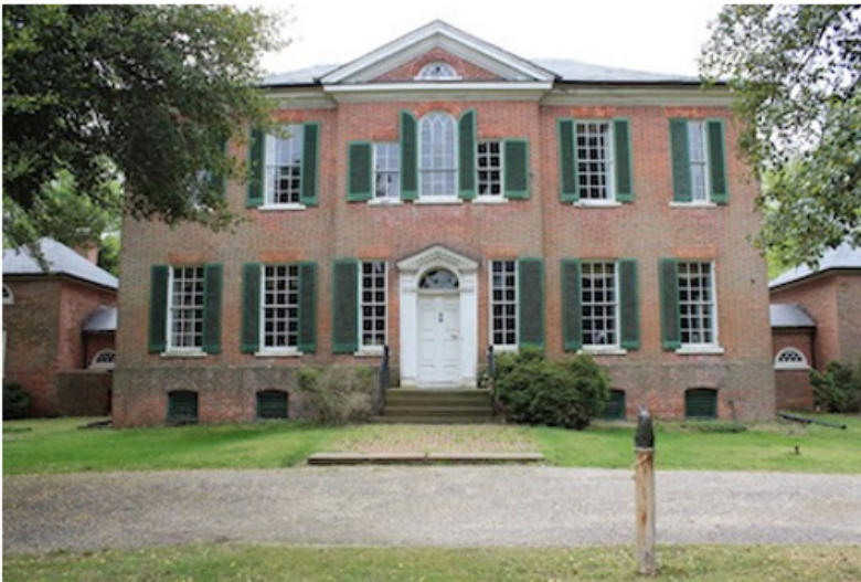
Photo 1 of 10: Front Façade, camera facing southeast.
