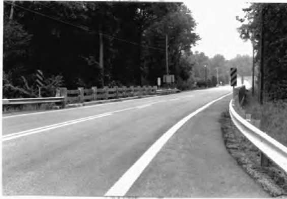
View of Bridge 1802000 (MHT, 1997).
