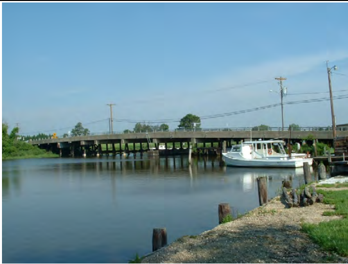
View facing south side of Bridge 0901600 (MDOT SHA, 2003).
