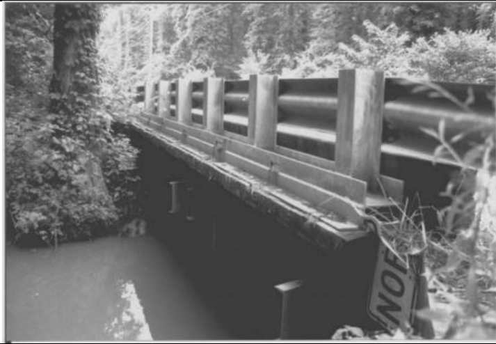
North elevation of Bridge 0402300 (MHT, 1997).
