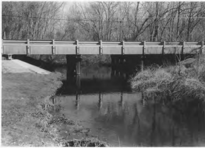
View, facing upstream, of Bridge 0900200 (MHT, 1998).
