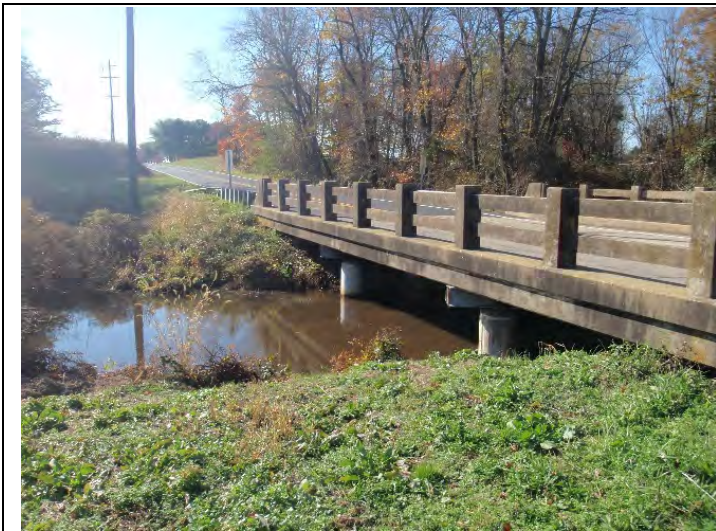
View showing concrete rails and pile jackets (MDOT SHA, 2013) .
