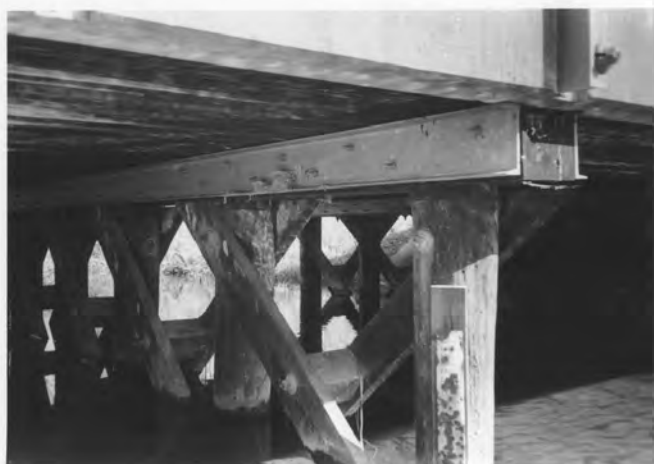
Detail showing timber stringers and galvanized pier cap (MHT, 1998).
