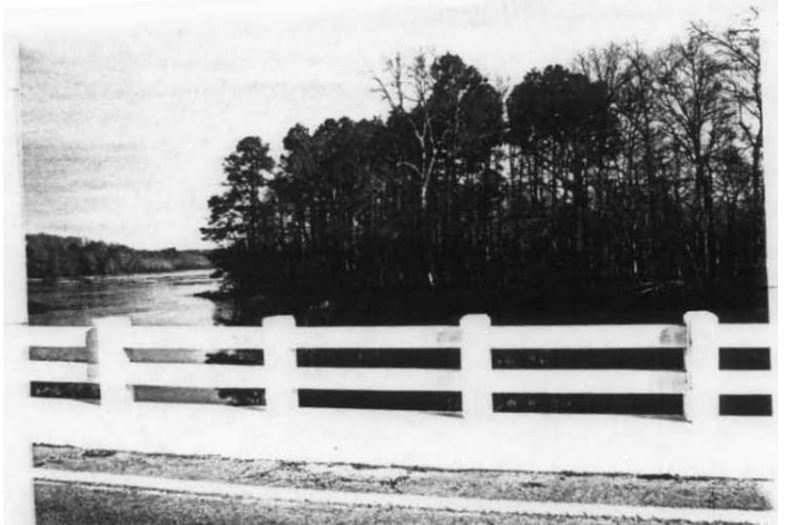
Facing north along Bridge 0900600 (MHT, 1993).
