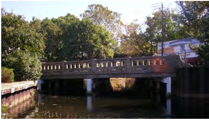
View facing east towards Bridge 2200400 (MDOT SHA, 2006).
