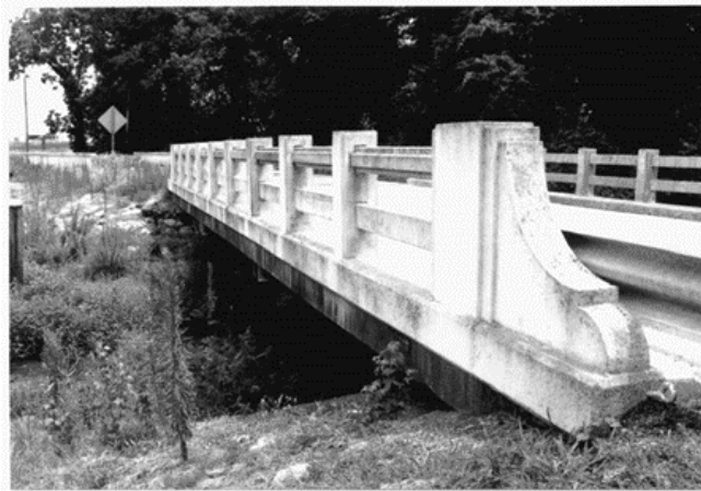
Detail showing concrete rail and Cyma-curve endposts (MHT, 1999).
