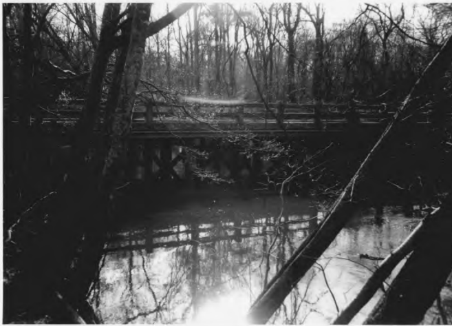
View facing downstream towards Bridge 2301700 (MHT, 1998).
