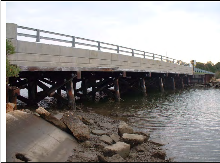
View facing south side of Bridge 1901300 (MDOT SHA, 2000).
