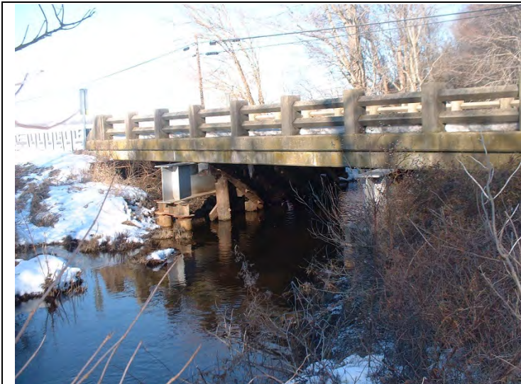
View of south side of bridge (MDOT SHA, 2000).
