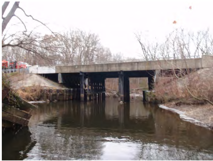
View of north side of Bridge 1703800 (MDOT SHA, 2008)
