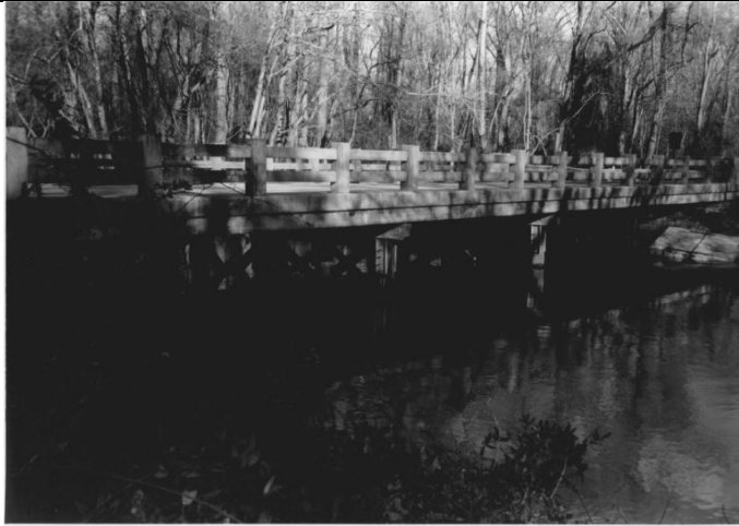
View facing upstream towards Bridge 2301700 (MHT, 1998).
