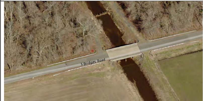
Birds-eye view, facing north, of Three Bridges Road over Burnt Mills Branch.
