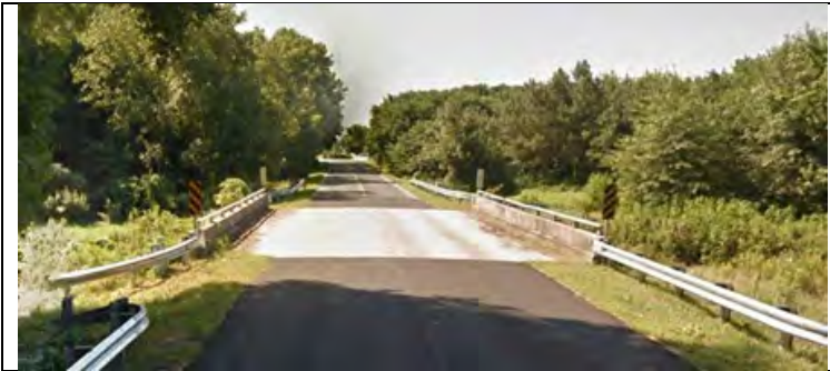
Facing south on Bethel Road towards Wicomico County Bridge WI-1661001 (Google Earth, 2014).
