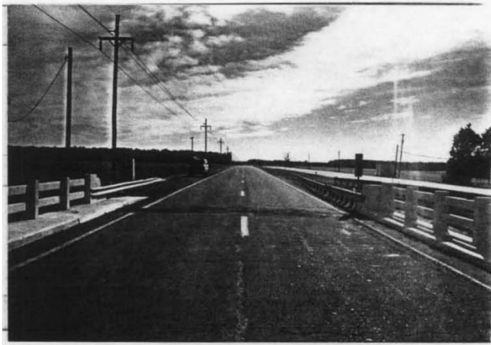
Facing east at east end of Bridge 0900600 (MHT, 1993).
