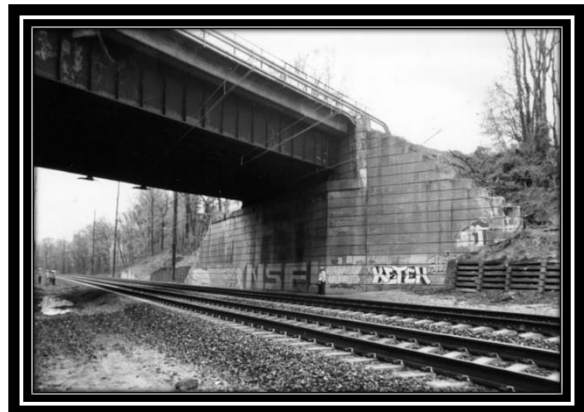
Figure 15. B&O Railroad Bridge over the B&P Railroad.
