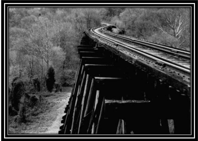
Figure 20. B&O Bridge over Antietam Creek, Long Bridge.
