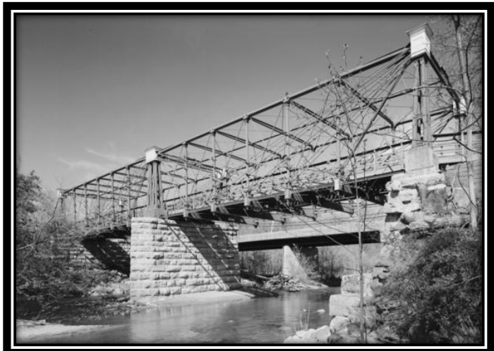
Figure 21. B&O, Bollman Truss Bridge, Savage, MD.
