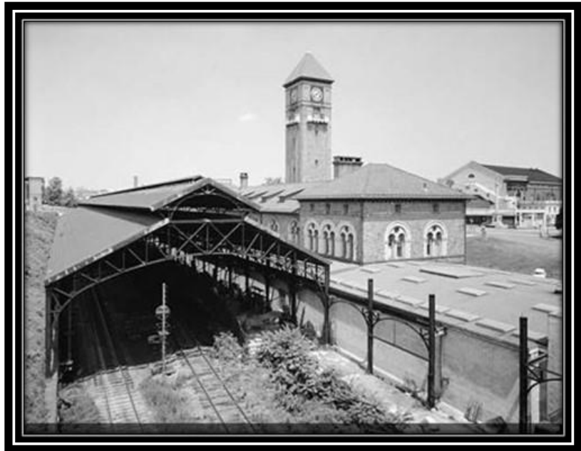
Figure 19. Mount Royal Train Shed, Baltimore, Maryland.
