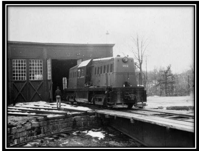
Figure 23. Chesapeake Beach Railroad Engine House and Turntable.
