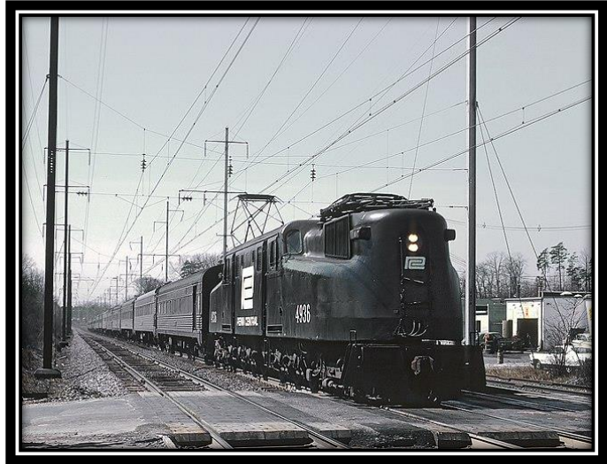
Figure 1. Catenary lines in use on the Silver Star at Seabrook, MD
